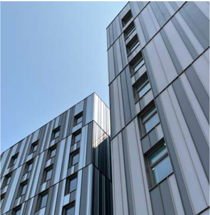
Facade: Stickbuilt Rainscreen
