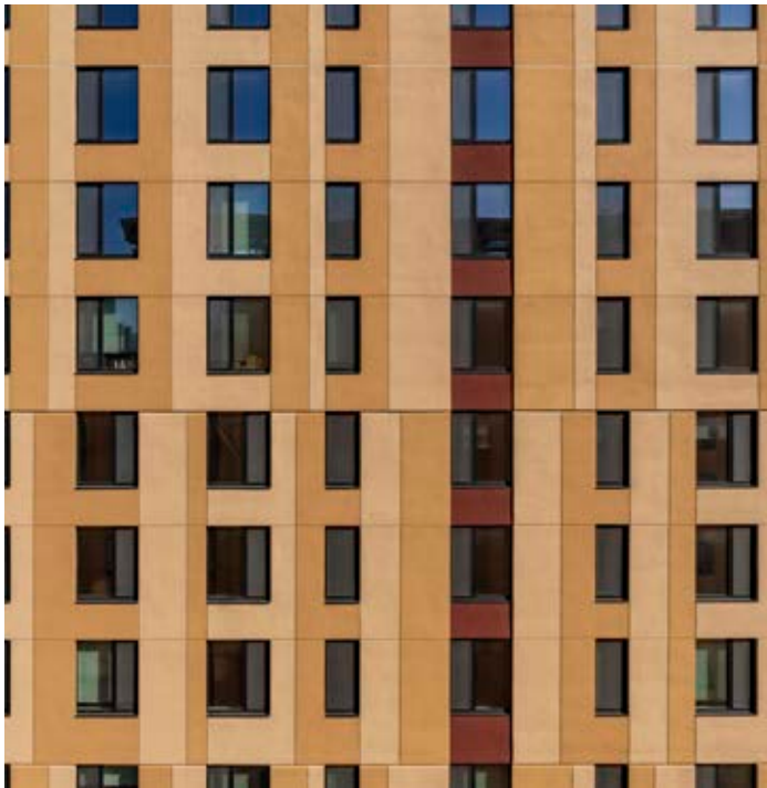
Facade: Masonry Cavity Wall & EIFS
