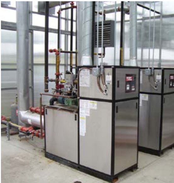
High-efficiency condensing boilers
