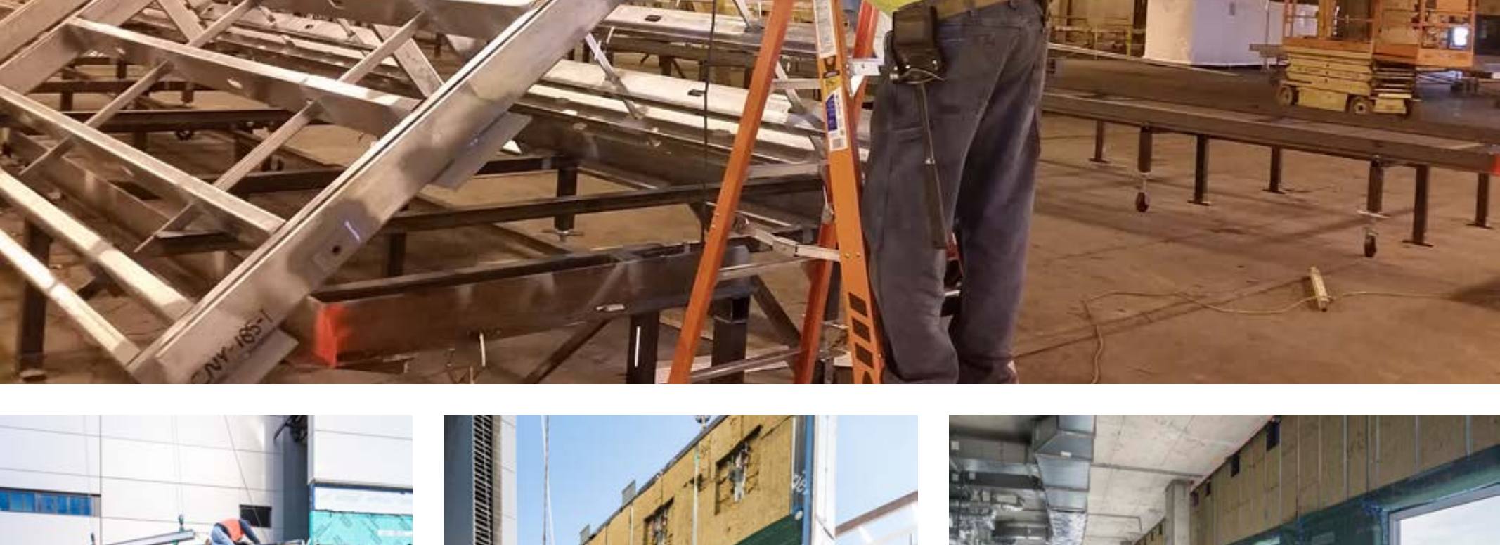
DIAGRAM Installing Prefabricated Panel Wall
