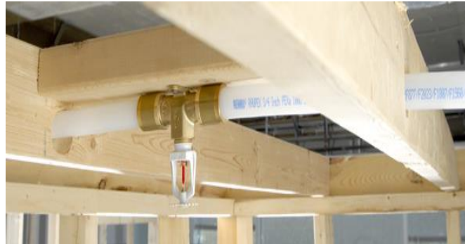
Low cost Plumbing integrated fire sprinkler components
