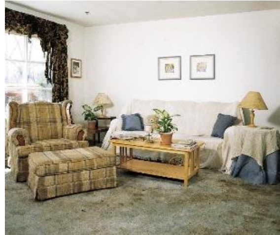
Living room protected by residential sprinklers
