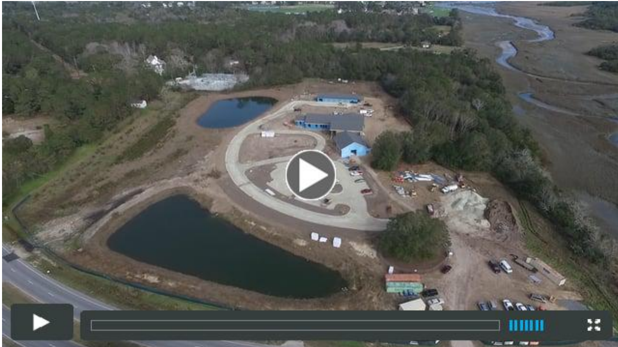
Kiawah Municipal Center Construction Video 19
