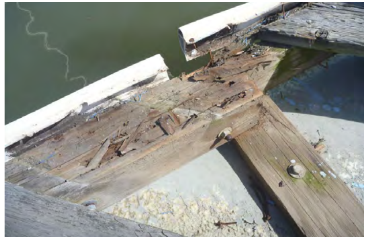
Dock D Finger Framing Structure - Broken deck boards and uneven walking surfaces
