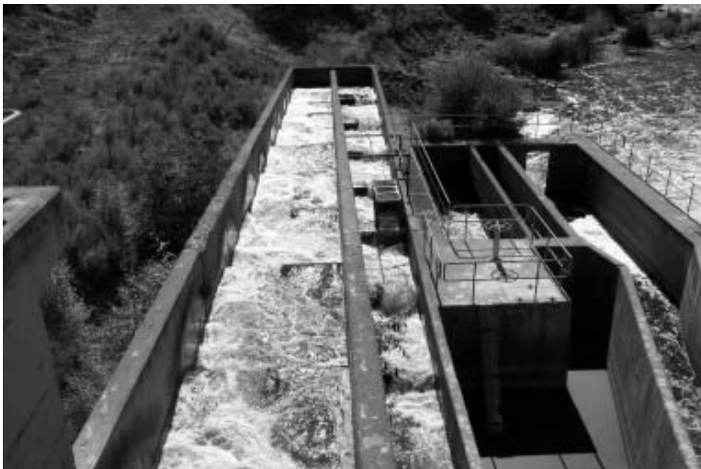
Photograph 1: Keno vertical slot fish ladder.
