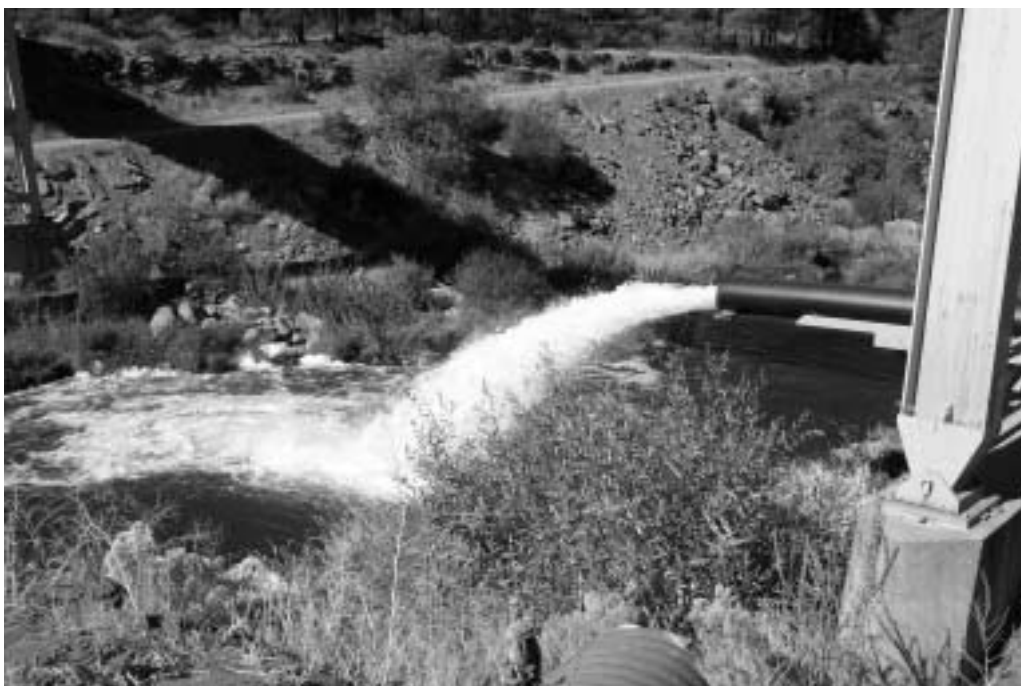
Photograph 3: JC Boyle bypass reach minimum flow and downstream migrant release pipe.
