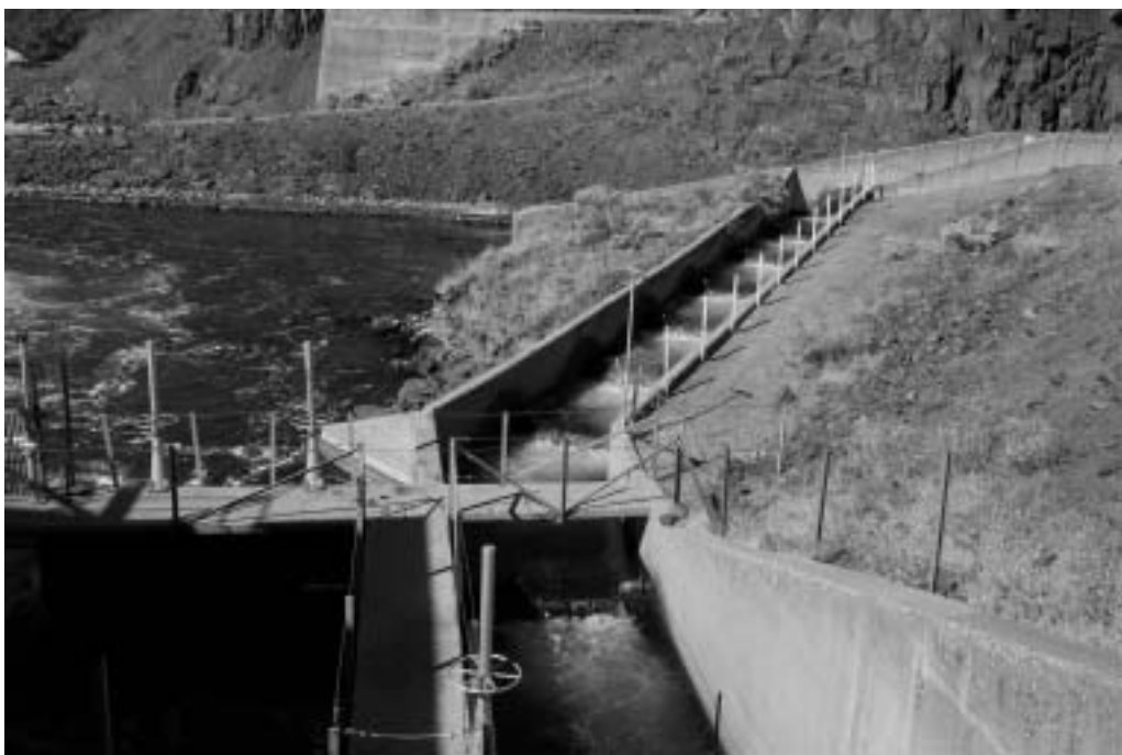
Photograph 6: Iron Gate pool and orifice ladder to fish holding ponds.
