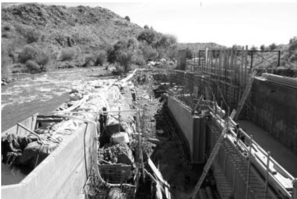
Photograph 4: New fish ladder construction at BOR's Link River Dam.
