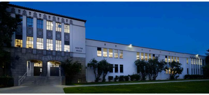
Originally built in 1937, South Hall is a three-story, 59,907 sf classroom building which required a complete modernization of the interior, voluntary seismic improvements including new footings and shotcrete shear walls, new electrical infrastructure, windows, suspended acoustical ceilings, restrooms, fire alarm, LED lighting, audio/visual, and ADA upgrades. Today's building codes and educational program needs differ markedly from those in the 1900's!
