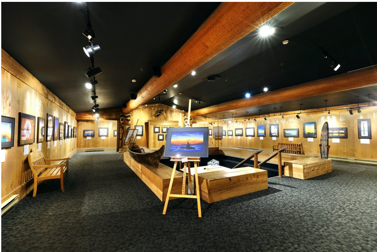
All the wood used in the construction of the gallery was found in Clayoquot Sound, for eg. the two old growth fir beams were sourced from an island in Kennedy Lake. Henry Nolla hand adzed every single cedar plank on the interior walls.
