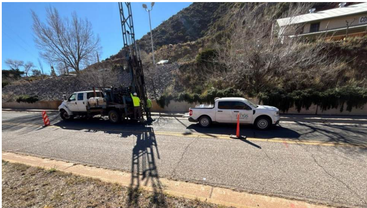
Photo 1: View of Boring B-2 Looking South
