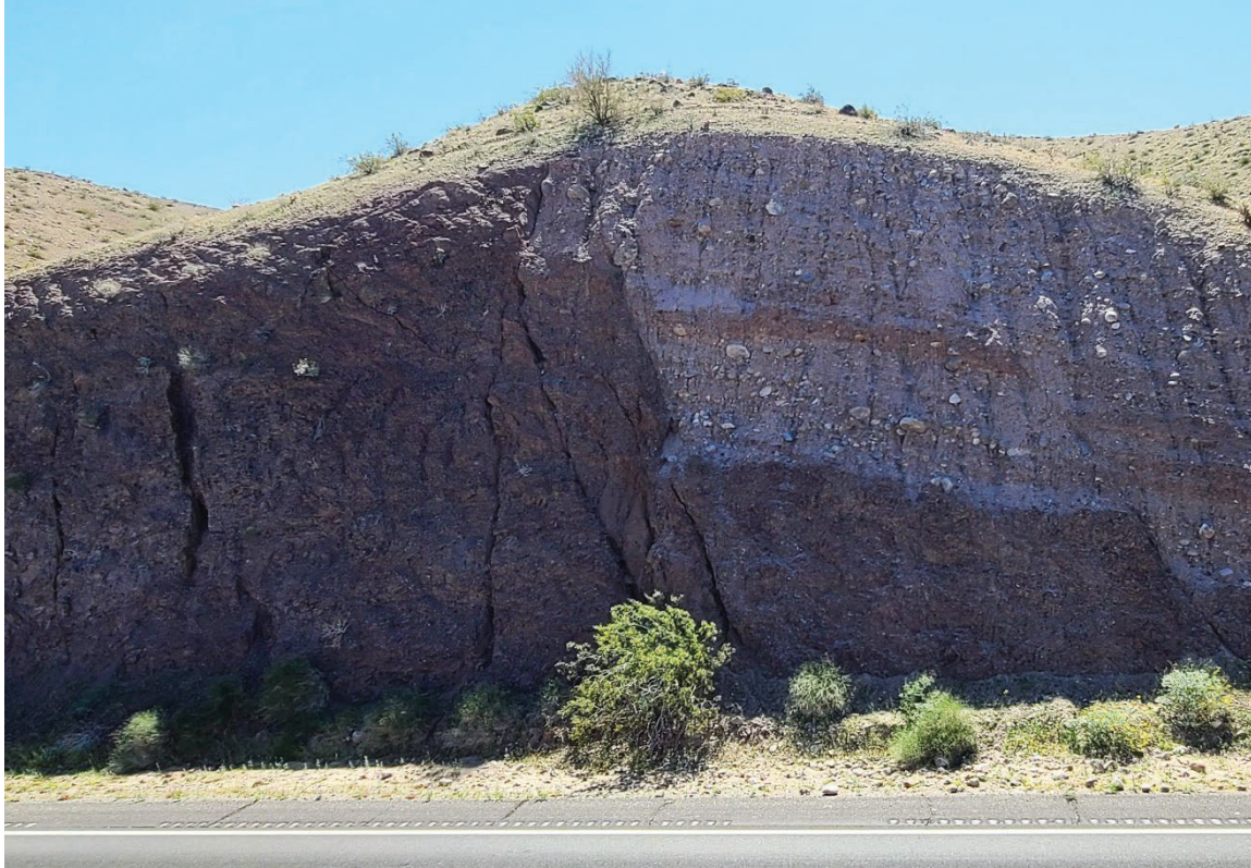
Figure 3: View of the cut slope along NB travel lanes at the location of SL-2
