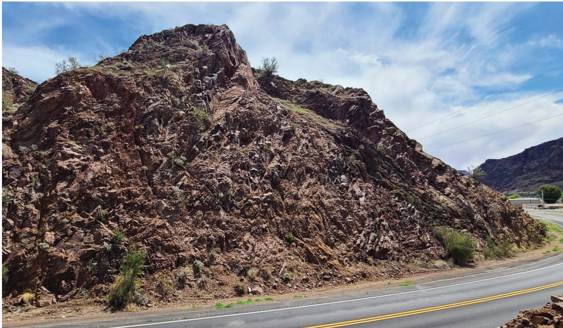
Figure 2: View of the cut slope along NB travel lanes at the location of SL-1
