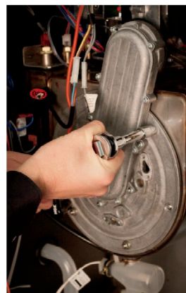
Re-install Gas Valve/Fan/Burner Plate
