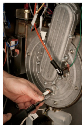
Re-install Flame Sensor
