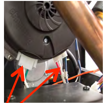
Remove 2 Molex Connectors (K2 5:1 model shown)
