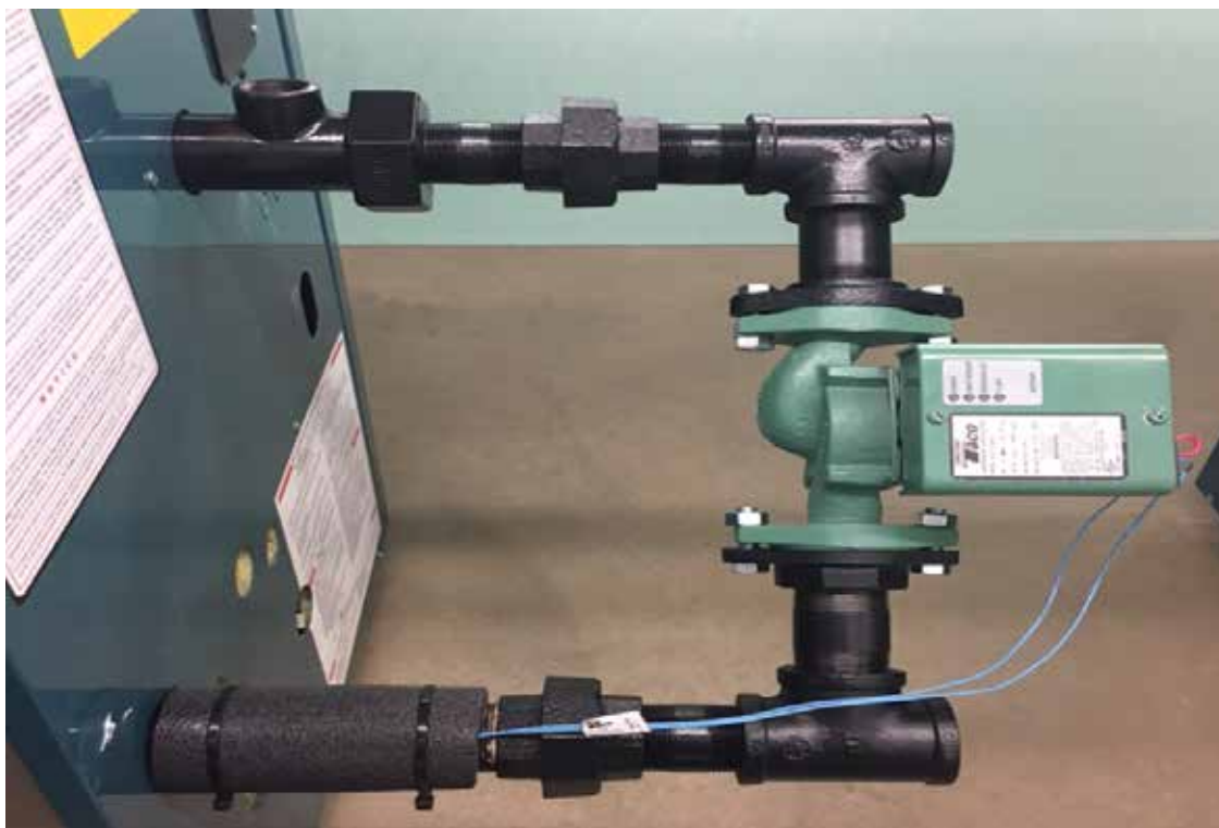
Figure 4 “Insulated Return Water Temperature S3
