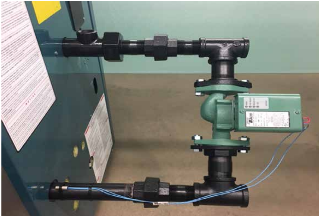
Figure 3 “Return Water Temperature S3 Strapped To Boiler Return Pipe Nipple
