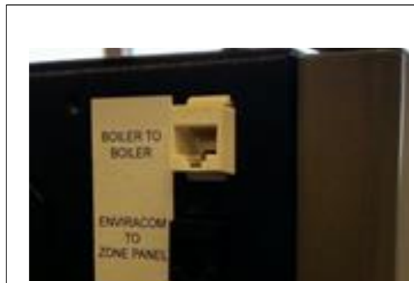
Figure 3-8: RJ45 Boiler to Boiler/EMS RJ45 Communication Port on Side of Boiler
