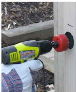
Drill hole in downspout
