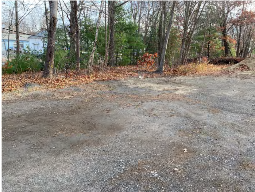
Figure 4. Low point where water is collected from Sudbury Lumber at approximately STA 701+00, facing northerly.
