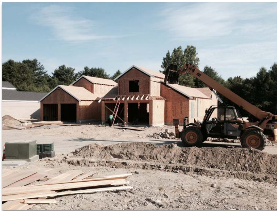
Left: Construction of a new home at Dudley Brook Preserve.
