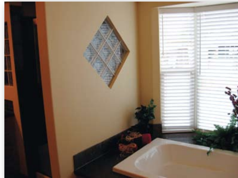
Decorative glass blocks in shower stall adding natural light into shower and a touch of elegance to the appearance of the bathroom
