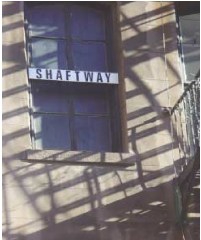
(Fig. 2.26) Exterior shaftway marking.
