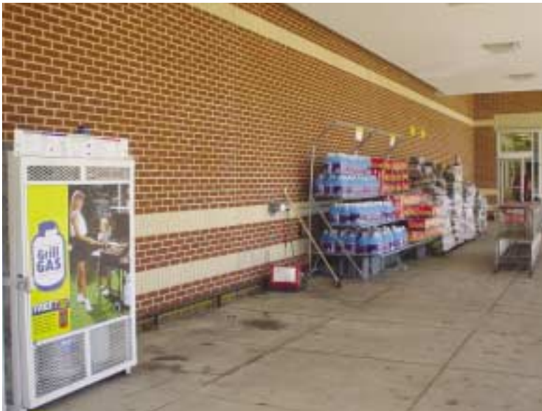
(Fig. 5.7) FDC in the cart area of a supermarket entryway. The FDC is located where merchandise or shopping carts could easily block it, or a fire in the adjacent propane storage area could restrict its use.
