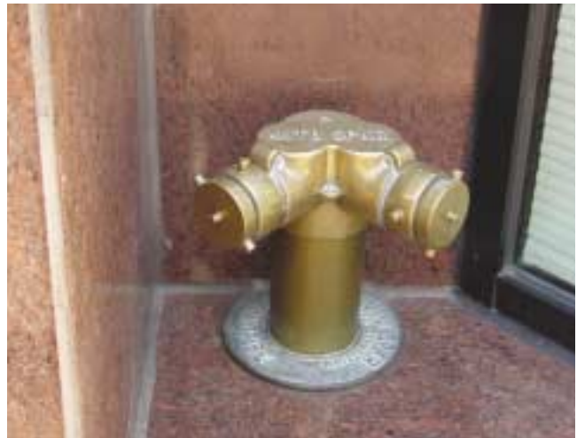
(Fig. 5.6) This FDC is mounted too close to a wall. Other obstructions could be fences, pipes, downspouts, vegetation, etc.
