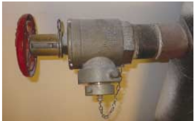
(Fig. 4.10) Hose connection equipped with a pressure regulating device.
