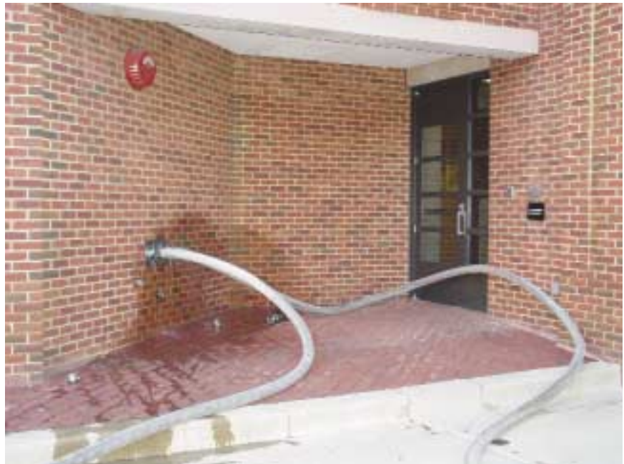
(Fig. 5.1) Charged hose lines connected to a wall-mounted FDC. The proximity of an FDC relative to building exits is discussed in the Location section at page 44.
