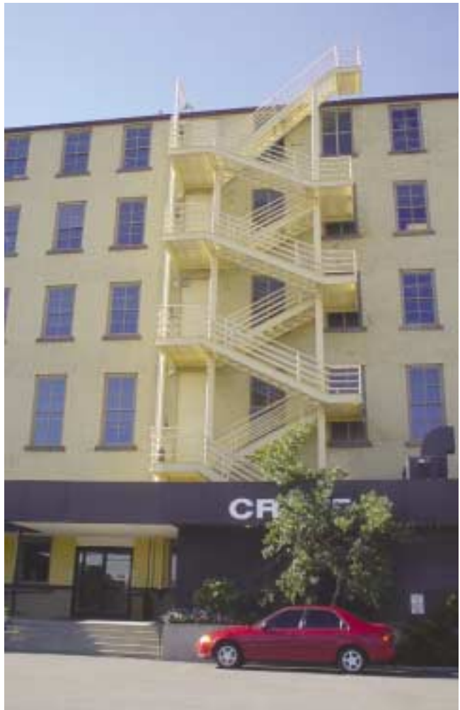
(Fig. 4.1) A dry standpipe in an exterior stair. The FDC inlet is to the right of the building entrance, the riser pipe extends through the left side stair landings, and hose connections are at each level, including the roof.
