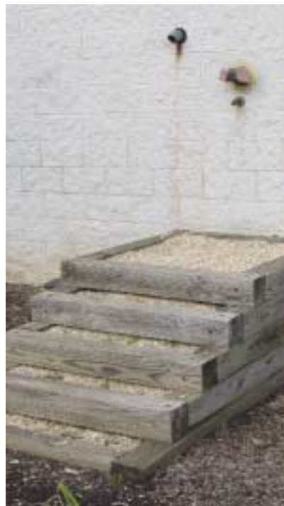
(Fig. 5.10) A platform built up to reach an FDC creates a hazardous condition. This should not be considered as equivalent to positioning the FDC at a proper height above grade level.
