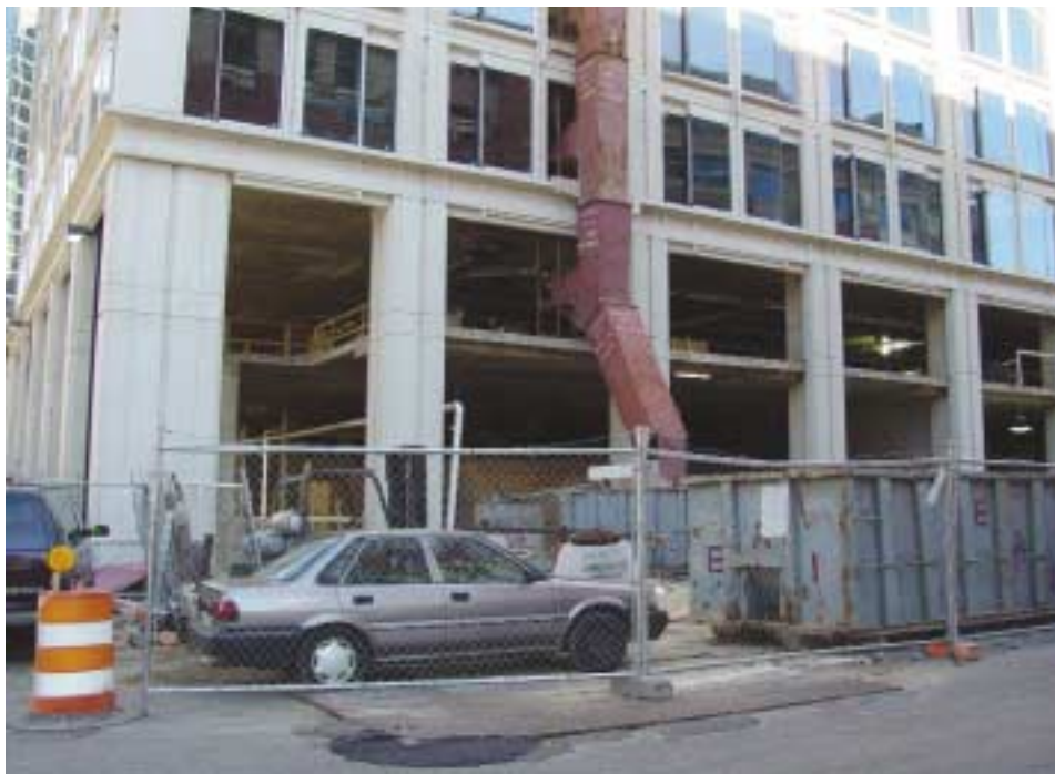
(Fig. 5.14) This is a building under construction as viewed from a piece of fire apparatus turning the corner onto the block. Can you see the FDC? It is not labeled, and it is blocked by a vehicle, a trash container, a fence, and construction materials. It is directly above the car's front bumper.
