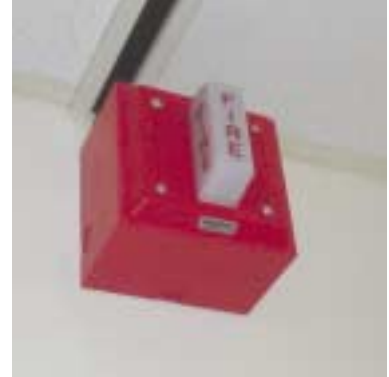
(Fig. 6.1c) Notification device (horn/strobe).
