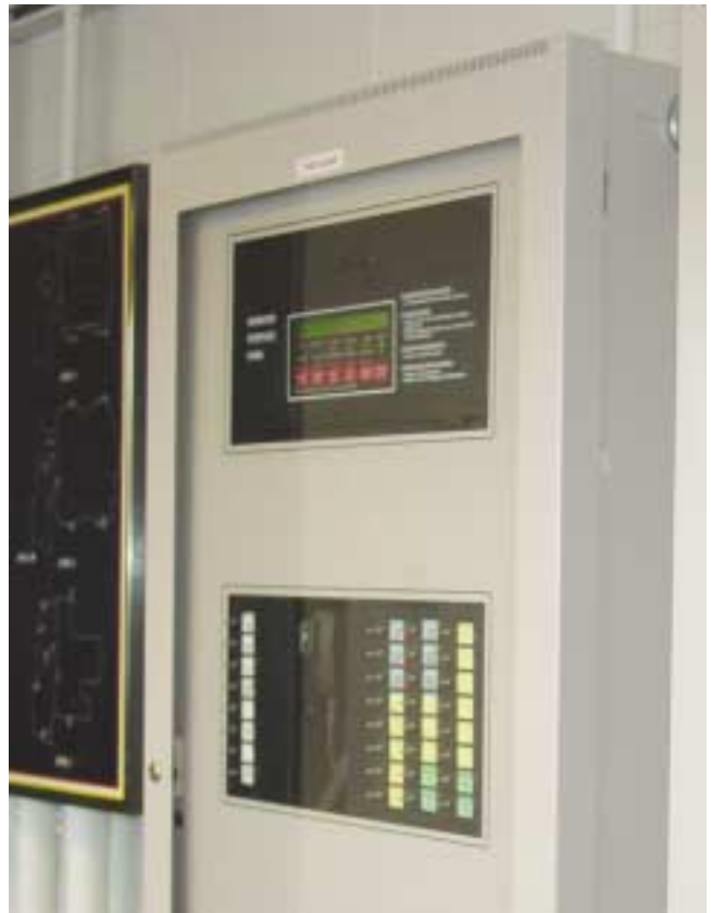
(Fig. 6.7) The grey panel is a voice alarm panel. The lower window shows the microphone and the manual select switches for the different evacuation zones.
