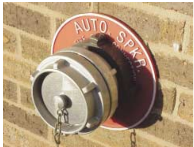
(Fig. 5.4) A quick-connect type of FDC.
