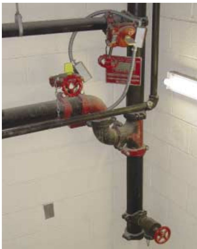
(Fig. 4.11) Isolation valve between the feed main (entering from the lower left) and the vertical riser (on the right). It is located within the stair enclosure for protection. The valve at the top of the photo is a sprinkler zone control valve.
