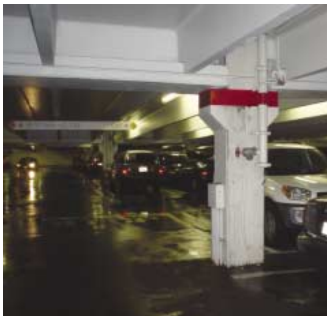
(Fig. 4.6) Stripe on column to identify hose connection location in a parking garage.
