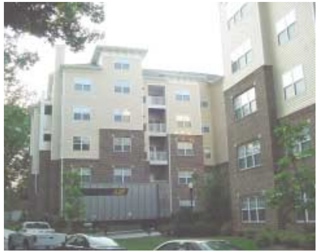
(Fig. 3.6) This building has six occupied levels from this view. However, it is classified as a four-story building by the code that was in effect during its construction. As such, an NFPA 13R residential sprinkler system (with no sprinklers in the combustibile attic or in the floor/ceiling assemblies) protects it.
