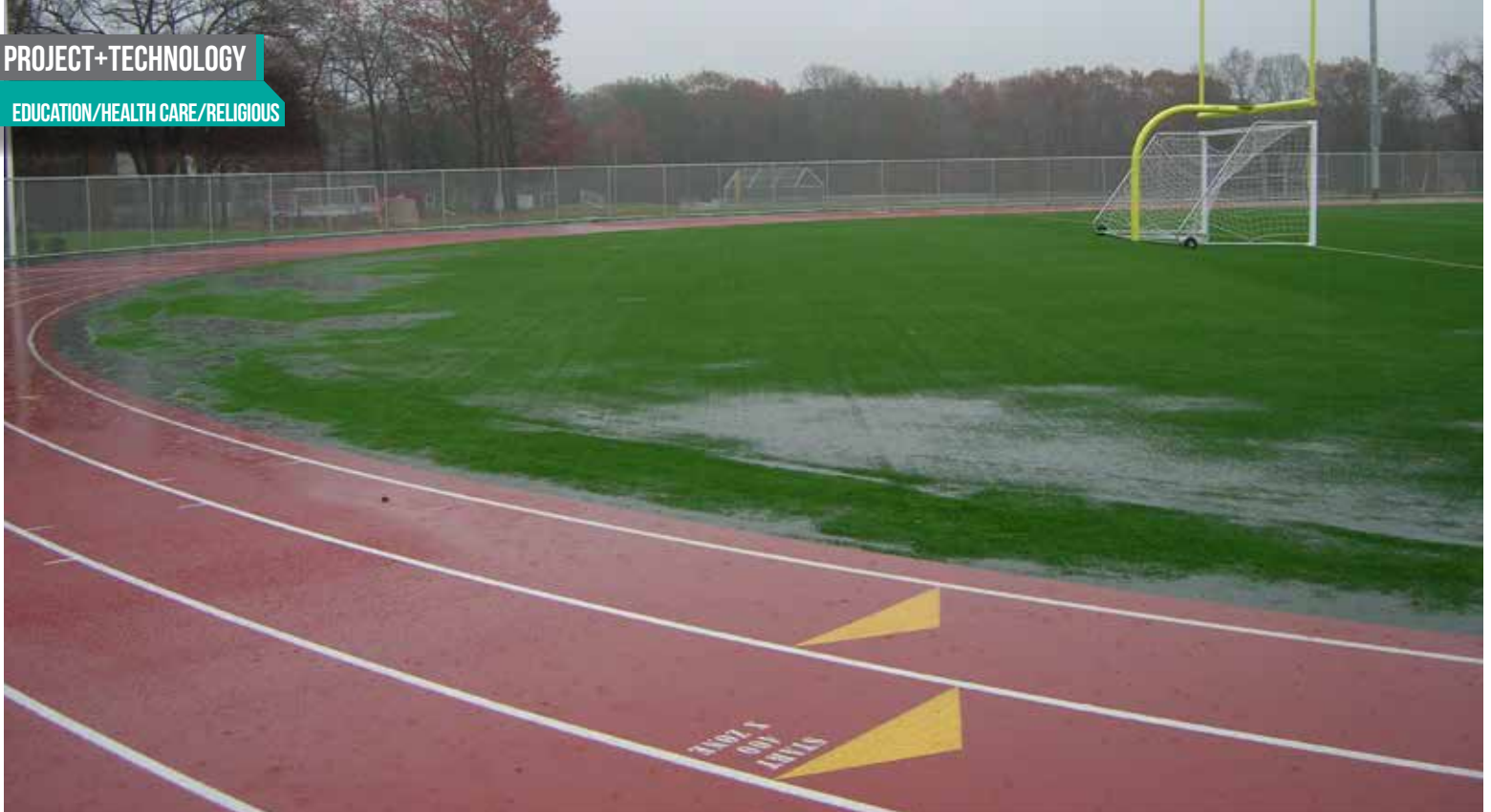
Figure 1: Ponding water on an artificial turf field. Photo: Town of East Greenwich, R.I.
