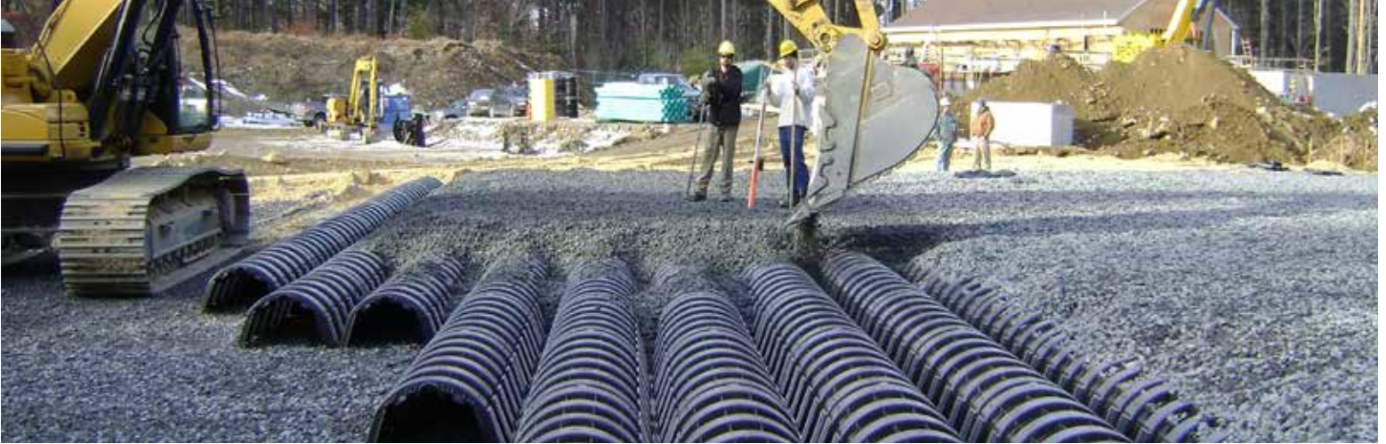
Workers backfill an 80,223-square-foot infiltration bed disposal field with a flow rate of 350,000 gpd at the Hopkinton, Mass. wastewater treatment plant.
