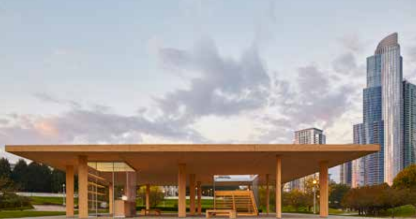
Chicago Horizon includes a cross laminated timber roof supported on 13 glulam columns distributed in a radial pattern to address lateral loads and uplift.
