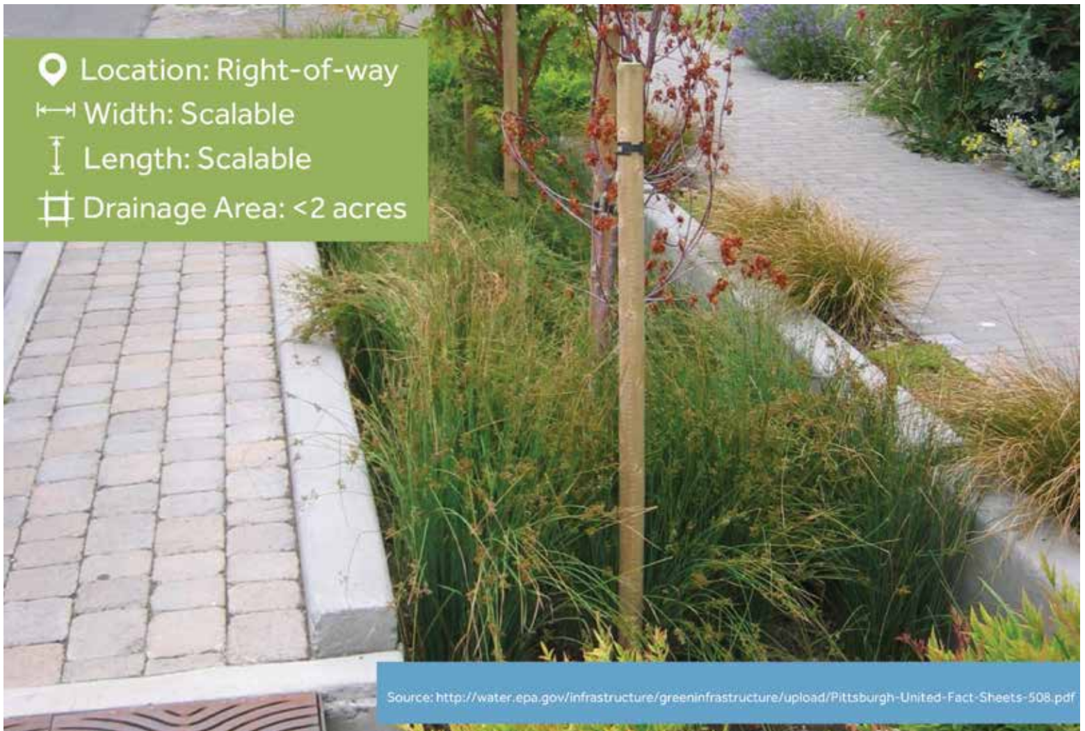
A stormwater planter is a linear infiltration basin that typically sits between a street and a sidewalk in the right-of-way and is surrounded by vertical curbing. Rainwater runoff flows to the gutter in the street and drains into the stormwater planter through openings in the curbing.
