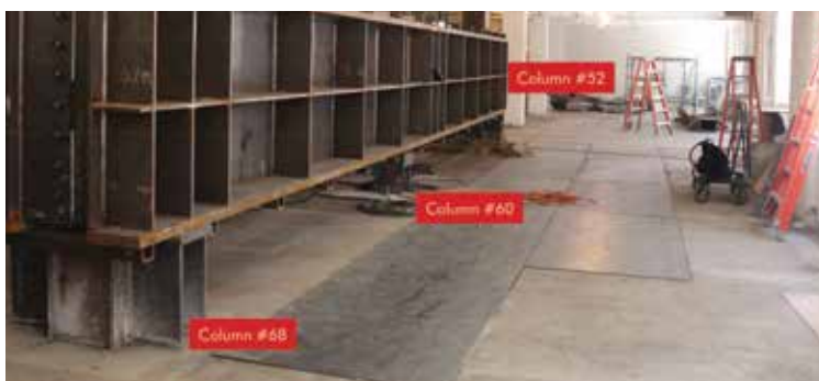
Figure 3: The transfer girder channel members were connected using stiffener plates and cross bracing at the top and bottom.
