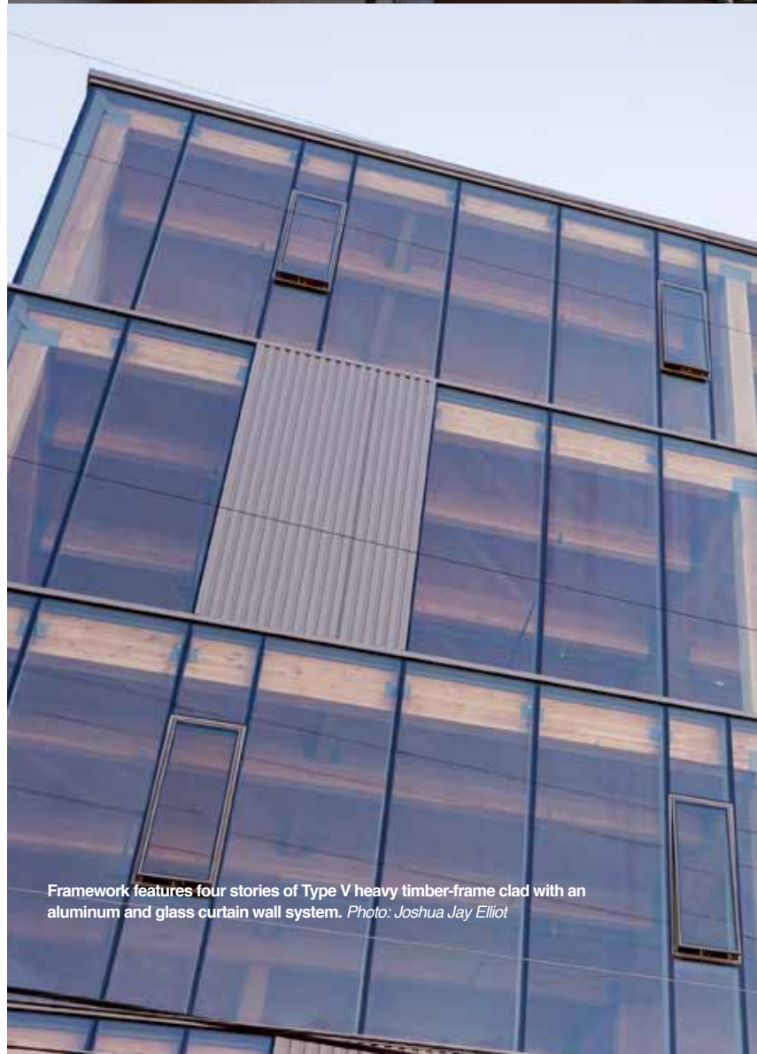
The Radiator’s gravity loads are handled through a system of glulam beams and columns. Thick timber decking creates the structural floor diaphragm. Photo: Caitlin Murry
