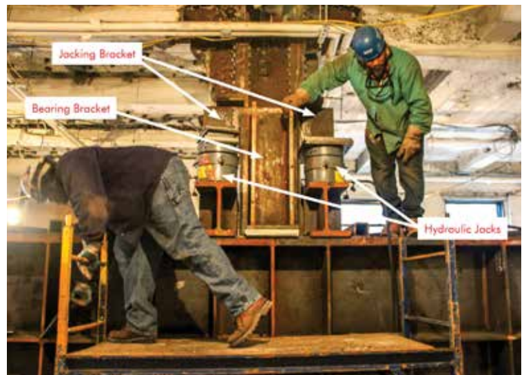
Figure 7: Two pairs of brackets were welded onto Column #60 — a pair of bearing brackets to transfer the load from the column onto the transfer girder and a pair of brackets used for jacking.
