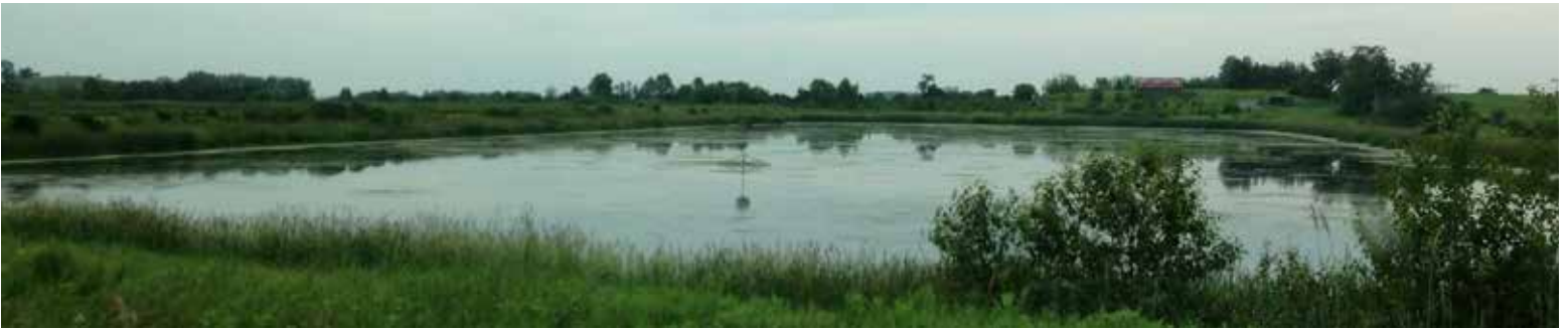
Benefits to the Village of Omeme, Ontario of a decentralized approach included that the town already owned the property, soils were well drained, and the lagoon-treated effluent was of a quality ready for disposal without additional treatment. Infiltration beds return water to the local aquifer, recharging groundwater supplies.
