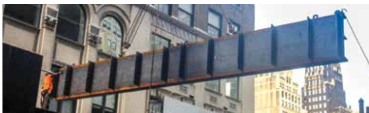
Figure 2: The transfer girder was designed as back-to-back built-up channels. The individual channel members were delivered into the building through a window on Level 2.
