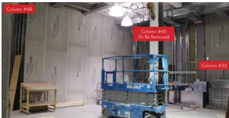
Figure 1: Column #60 (center) was removed between the first and the second floor.
