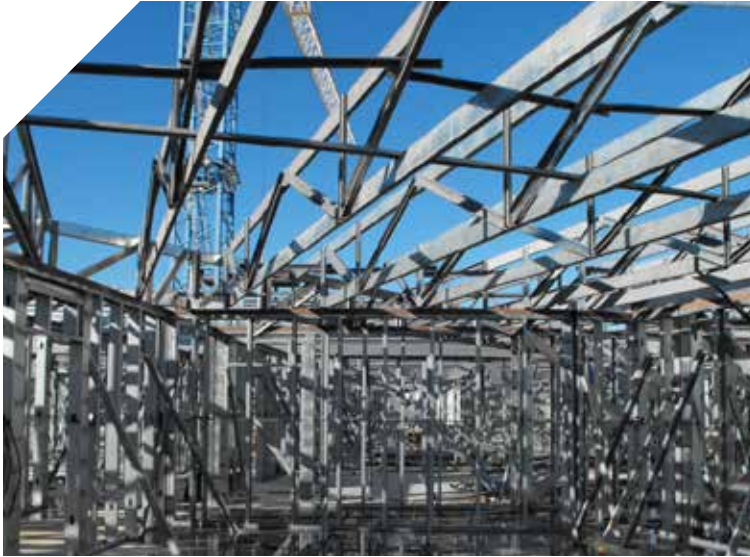
The Elan Westside roof was made up of pre-engineered cold-formed steel trusses. Photo: DSi Engineering
