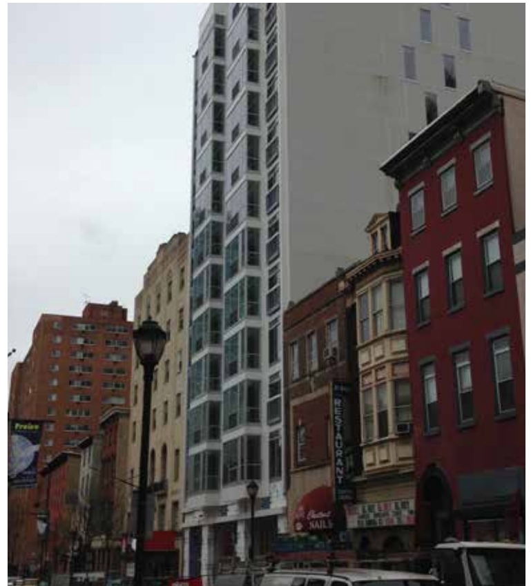
To accommodate a short construction schedule and tight quarters, external framing was panelized offsite with exterior sheathing and finishes applied. Photo: ClarkDietrich
