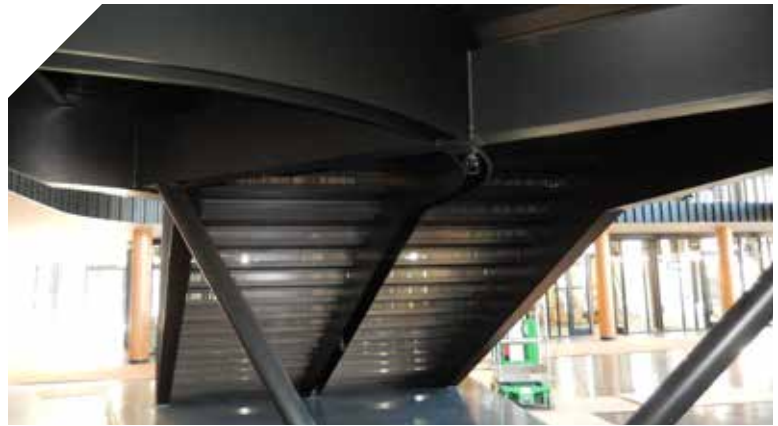
Peek-a-boo sprinkler heads with pipelines integrated within a central double fin plate stair stringer. Photo: © Arup/Jimmy Su
