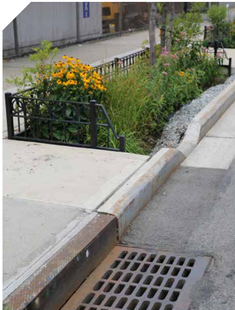
On average, across all three demonstration areas during a typical rainstorm in New York City, the green infrastructure reduced the stormwater runoff entering the sewer system by at least 20 percent. Photo: New York City Department of Environmental Protection
