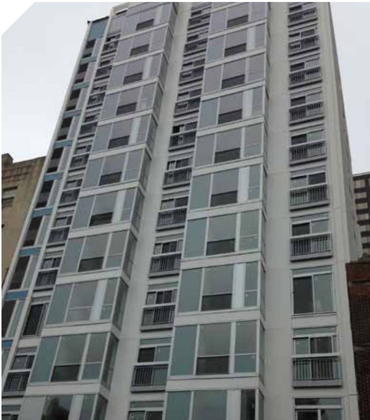
The AQ Rittenhouse luxury apartment complex features a structural steel frame, concrete slabs, and exterior cold-formed steel framing. Photo: ClarkDietrich
