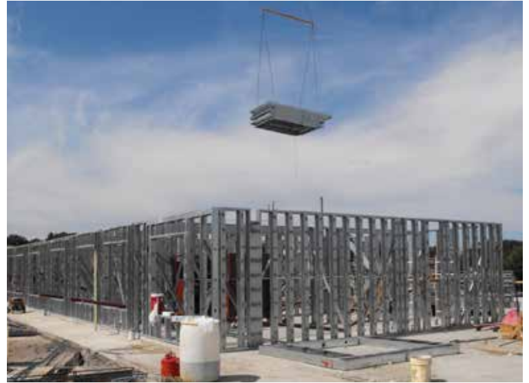
The Elan Westside project combined welded, pre-panelized load-bearing cold-formed steel walls, structural steel, and dovetail composite deck supporting a floor slab. Photo: DSi Engineering
