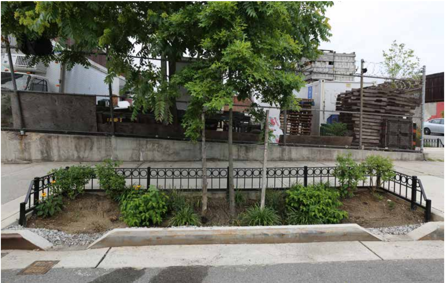
Bioswales resemble standard street tree pits, except that they vary in size, have curb cuts that allow stormwater to enter and overflow if it becomes saturated, and have been designed in a way that will allow them to manage between 1,100 and 2,200 gallons each during a storm. Photo: New York City Department of Environmental Protection
