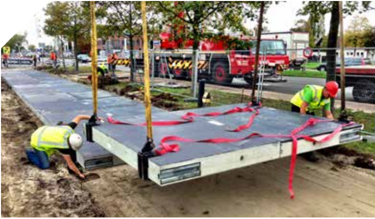
SolaRoad consists of a cycle path constructed of concrete modules with solar cells fitted underneath a tempered glass top layer that is covered by a transparent and skid-resistant coating.
