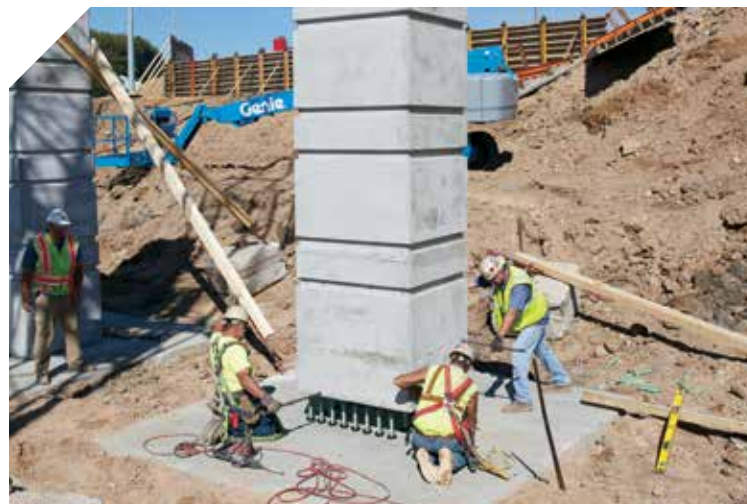
Precast bridge columns, girders, and pier caps allowed for faster bridge construction.
