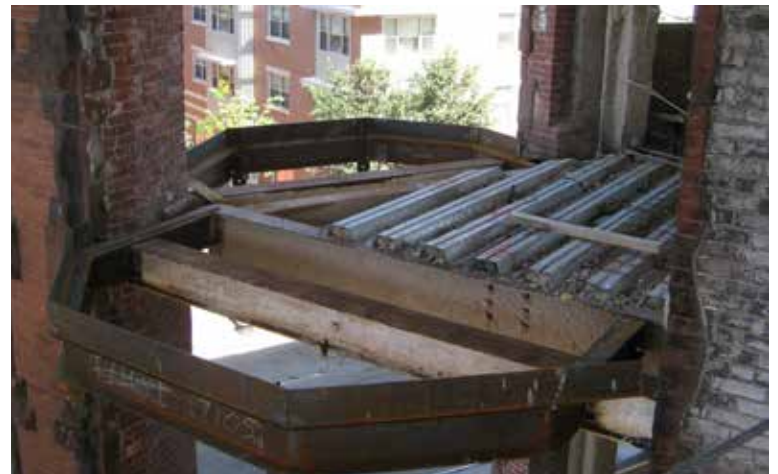
Steel framing to resupport cantilevered bay windows at the Curtis and Waterman façade. Photo: © Arup/Jimmy Su
