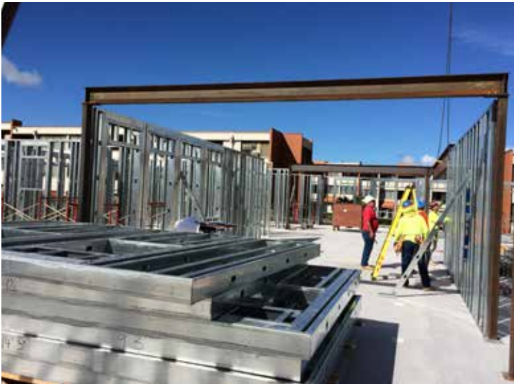
A load-bearing cold-formed steel system in combination with a framed floor system with Structo-Crete panels reduced the dead load of the structure compared with traditional building materials while maintaining a noncombustible classification up to the roof line. Photo: CEMCO
