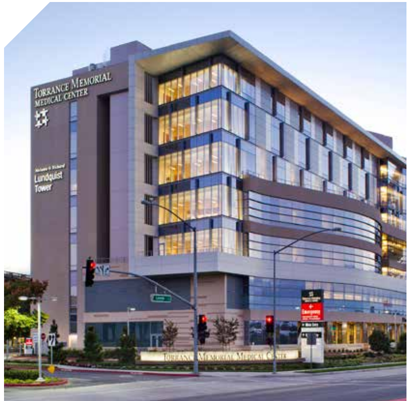
The Lundquist Tower's exterior skin is a combination of metal panel, precast concrete, plaster, and curtain wall. BIM 3D modeling aided in clash detection and coordination of the seismic bracing and exterior skin systems.
