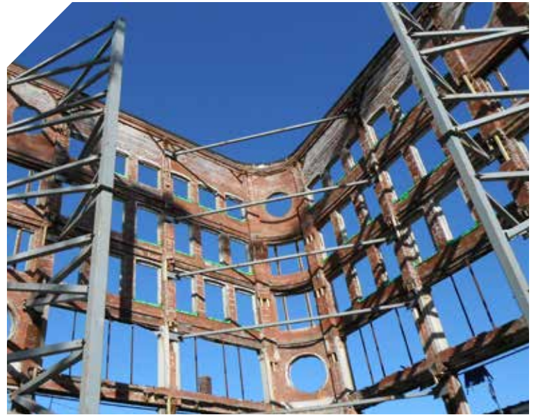
A view from the interior side of the Ferdinand façade after removal of all interior structure, with temporary supports installed by the contractor, coordinated with the incoming permanent structure. Photo: © Arup/Jimmy Su
