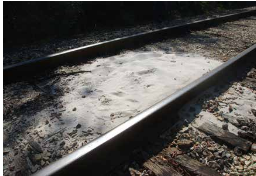
Fine grains of frac sand can leak from rail cars, accumulate in rail bed ballast and, during a rainstorm, turn into mushy, track-loosening mud. Photo: Tuncer Edil/UW-Madison
