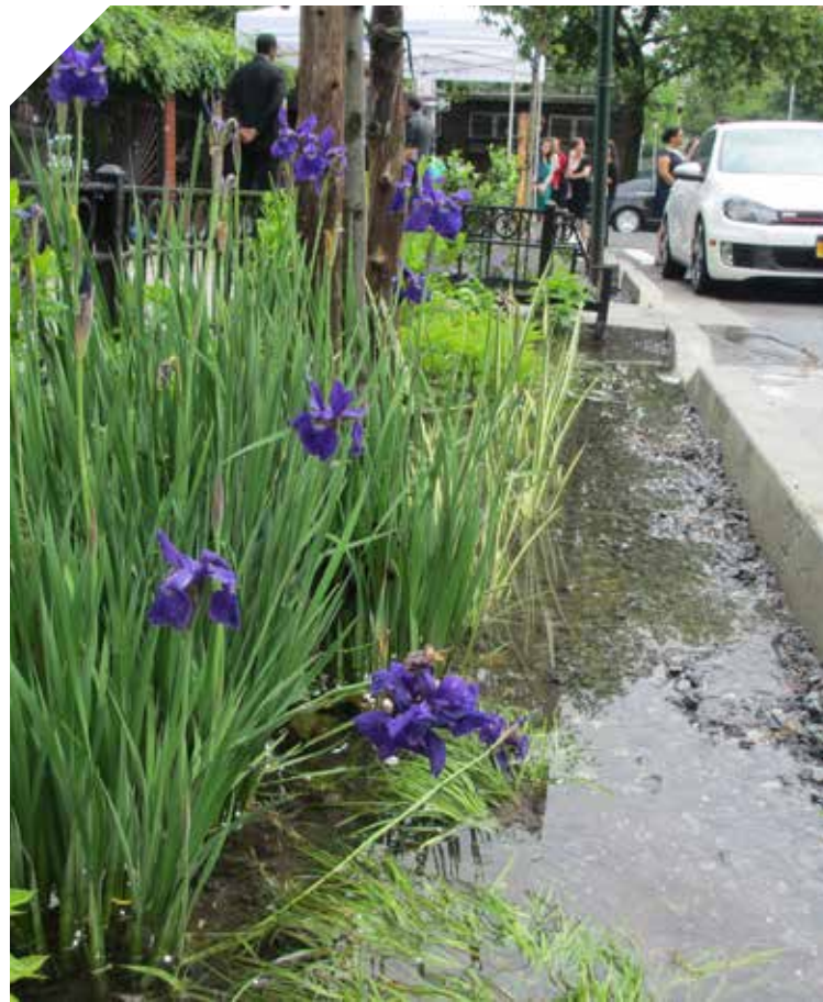
Inclusion of a stone gabion, which hydraulically connects the surface of the bioswale to the storage layer beneath the soil, helps to speed absorption of stormwater. Photo: New York City Department of Environmental Protection
