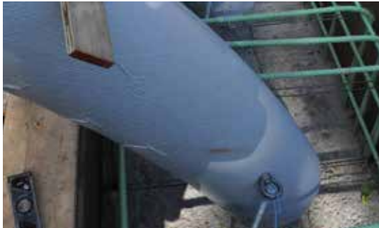
1) FRP arch tube units are secured to cast-in-place concrete footing rebar on both ends of the bridge
