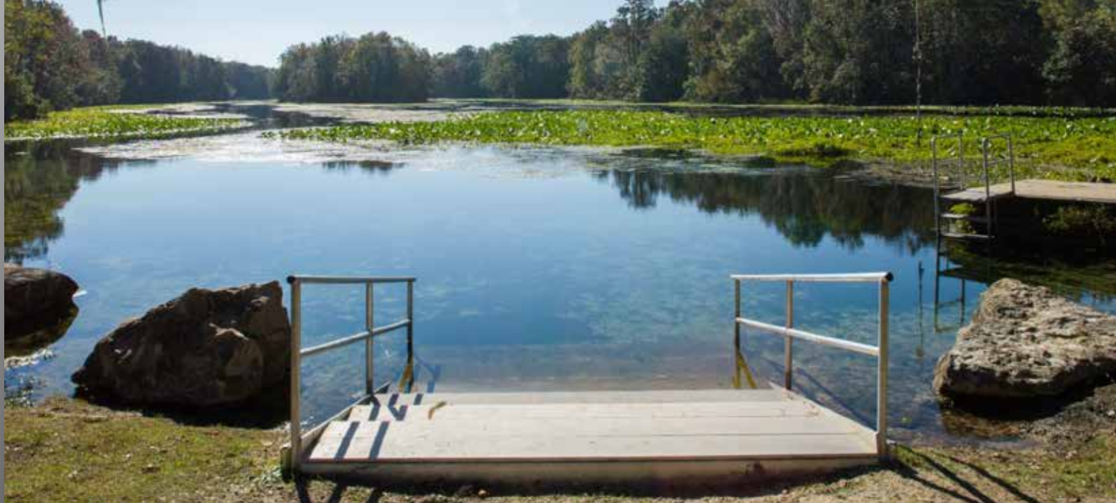
Swim ladders and stairs were installed to discourage swimmers from climbing on the shoreline to enter and leave the swimming area, stabilizing the spring banks to control erosion. Photo: Dewberry
