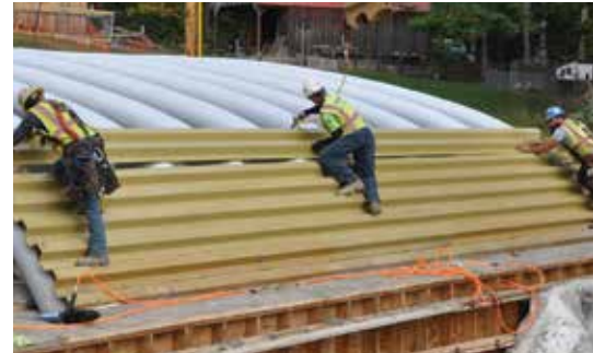
3) FRP decking is installed along the top of the arch units
