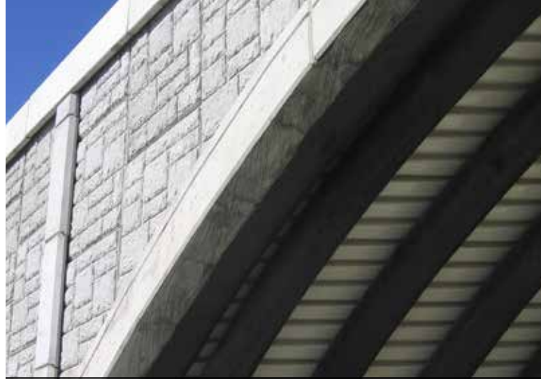
The 54-foot span Farm Access Overpass in Caribou, Maine, with a stone finish precast concrete MSE wall. Image: Advanced Infrastructure Technologies, Inc.
