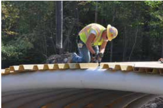
1) FRP arch tube units are secured to cast-in-place concrete footing rebar on both ends of the bridge
