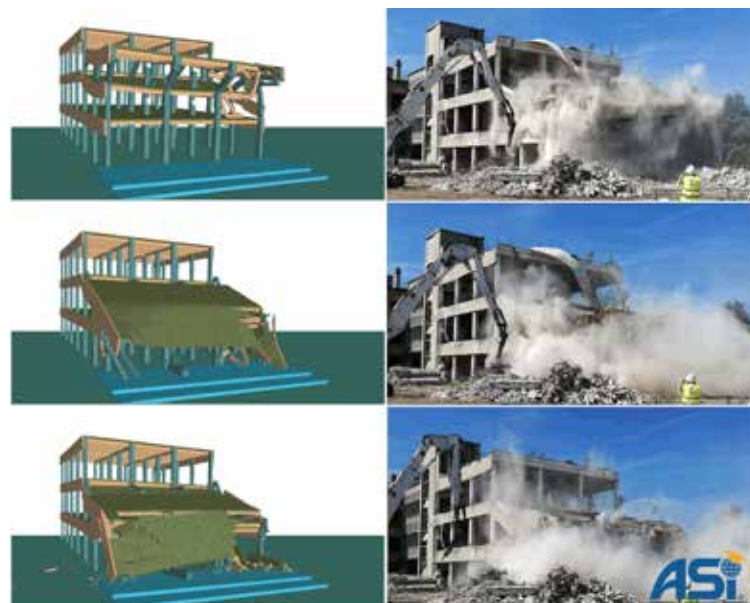
Frames from a video sequence of the actual collapse (right) and INACHUS collapse simulation software.
