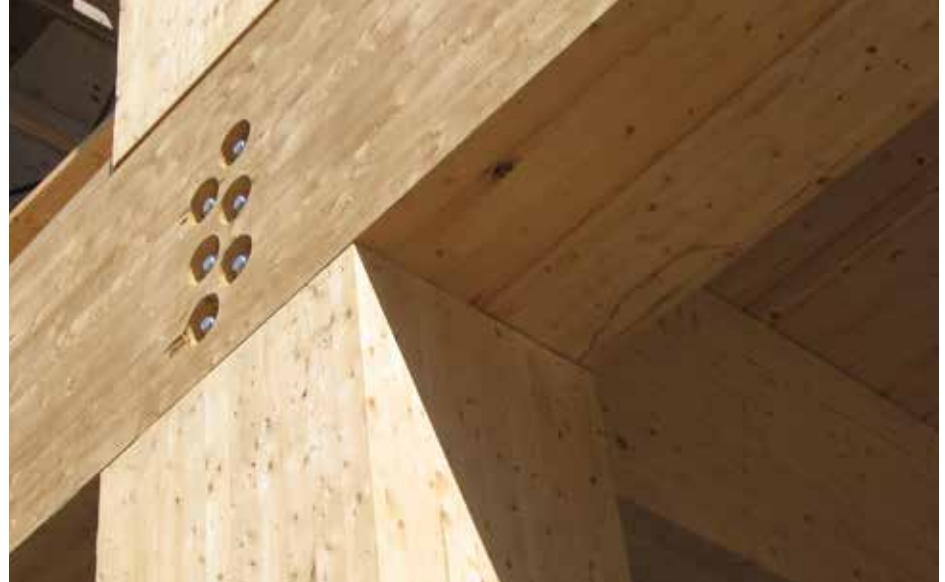
Mass timber — cross-laminated timber, nail-laminated timber, and glue-laminated timber — and wood has an appeal for multifamily low- and mid-rise construction. Photo: FPIInnovations
