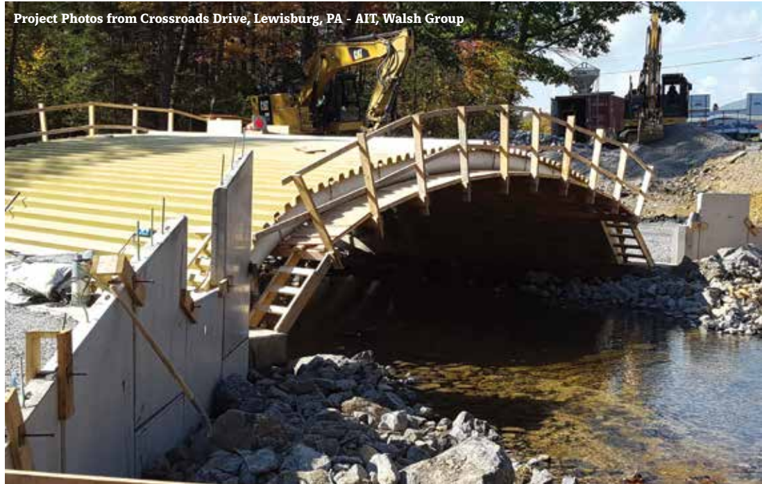
5) MSE spandrel walls and wing walls are installed to create the roadway grade
