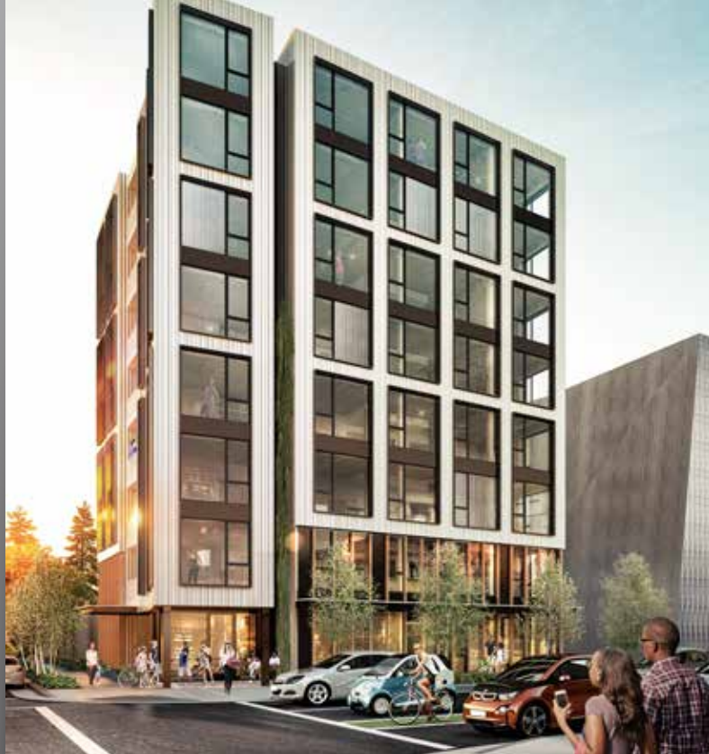
The eight-story Carbon 12 uses a hybrid system of cross-laminated timber floor and roof diaphragms and steel core. Image: Baumberger Studio
