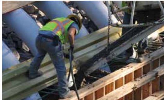
2) Cast-in-place concrete footings are poured
