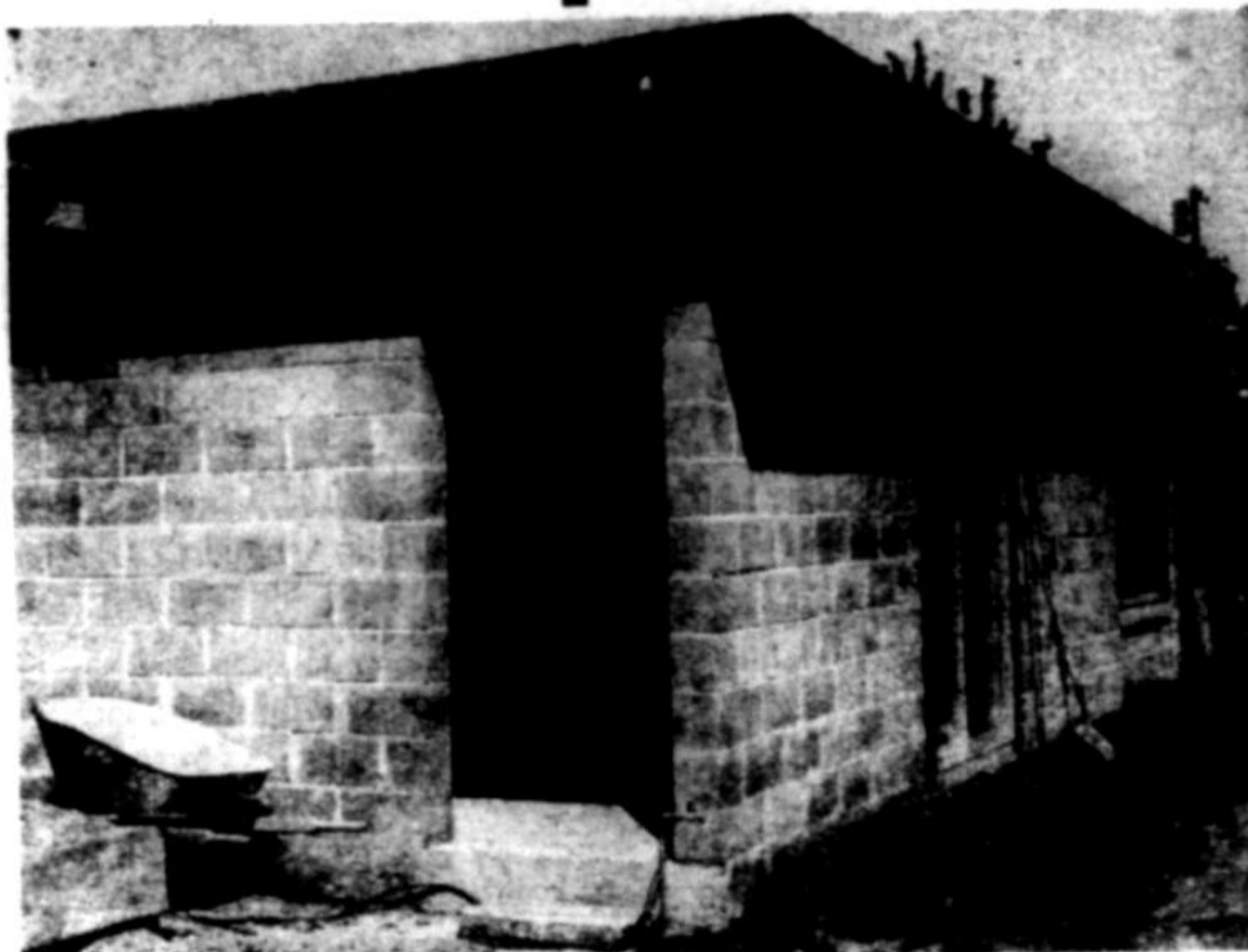
MEIKLEJOHN CIVIL RIGHTS LIBRARY Nearing Completion
