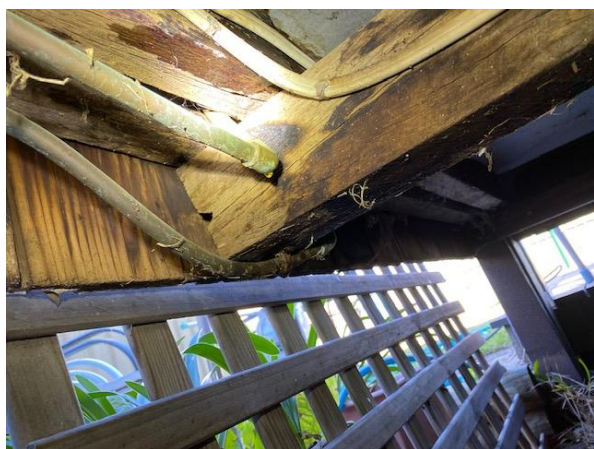
Leaking laundry tub below laundry in subfloor
