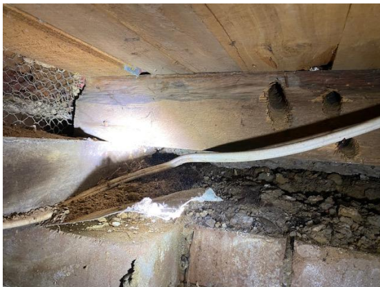
Timber Bearers in ground contact – inadequate termite protection
