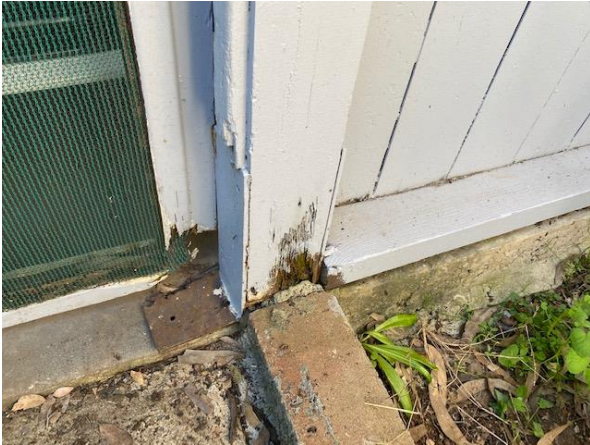
Wood rot present in carport timbers and around the property
