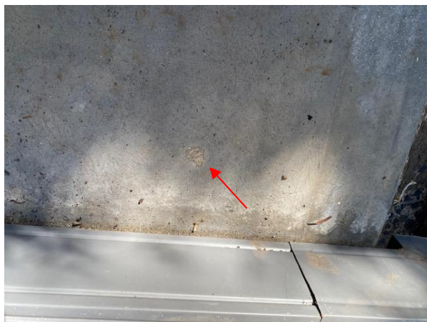
Drill holes in front veranda indicating possible previous termite treatment
