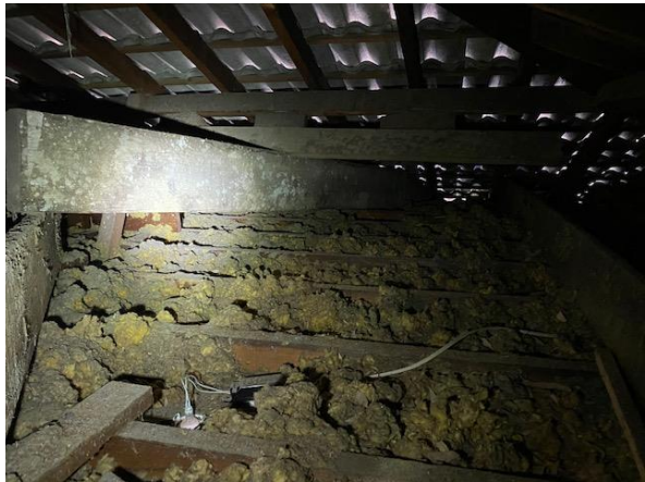
Insulation in roof void restriction inspection
