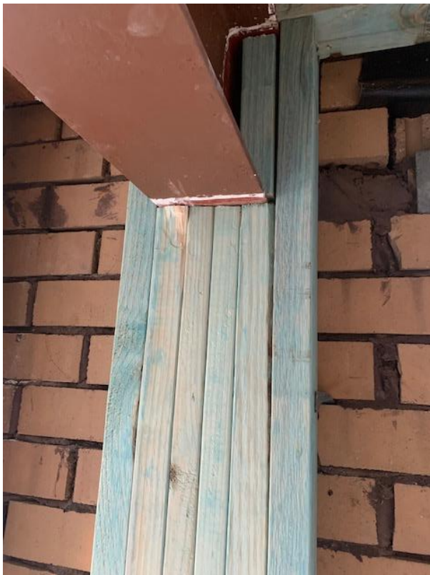
Rectified Termite Damage as at 14 th April 2021
