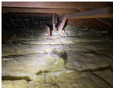
Insulation in roof void obstructing inspection zone
