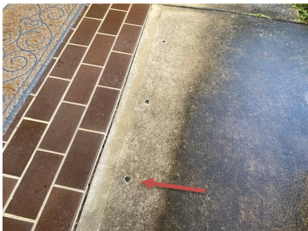
Drill holes located to the perimeter of the house
