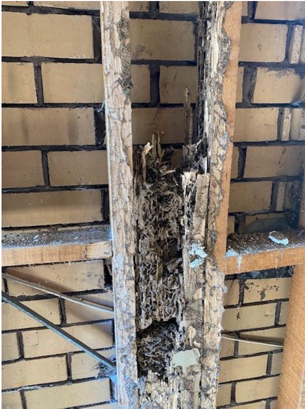
Previous Termite Damage at the time of Inspection.
