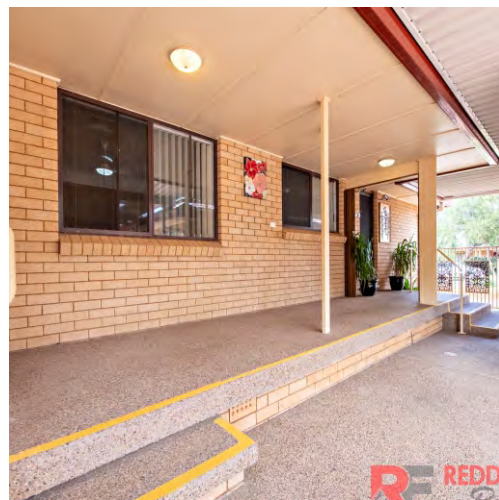
ELEVATED BACK VERANDAH
