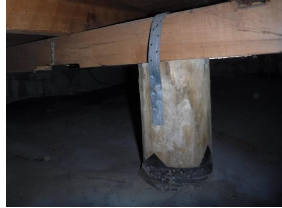
Photo 11. Sub floor space (View 1)
