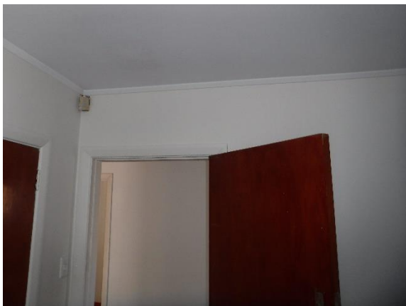
Photo 8. Dwelling wall lining and ceiling
