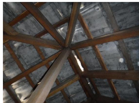
Photo 15. Roof space (View2)
