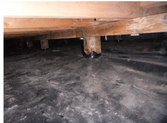
Photo 13. Sub floor space (View 3)
