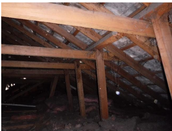
Photo 14. Roof space (View1)
