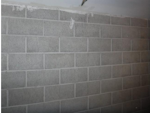
Photo 10. Garage concrete block wall from interior view.
