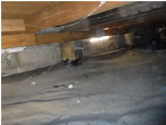
Photo 12. Sub floor space (View 2)
