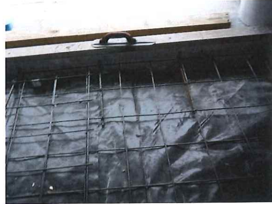
Photo 2. Garage concrete floor prior to pour concrete (View2)
