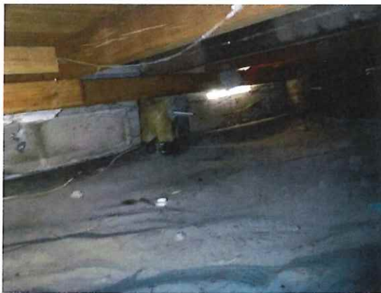
Photo 12. Sub floor space (View 2)
