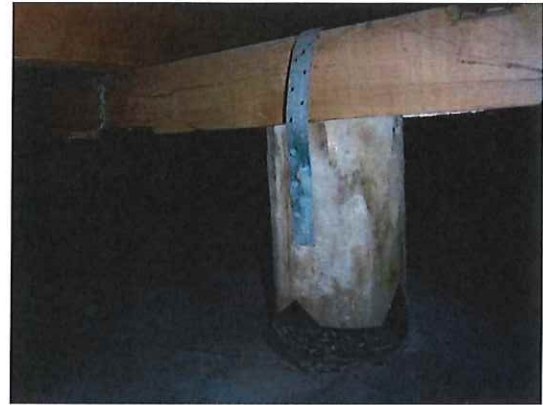
Photo 11. Sub floor space (View 1)
