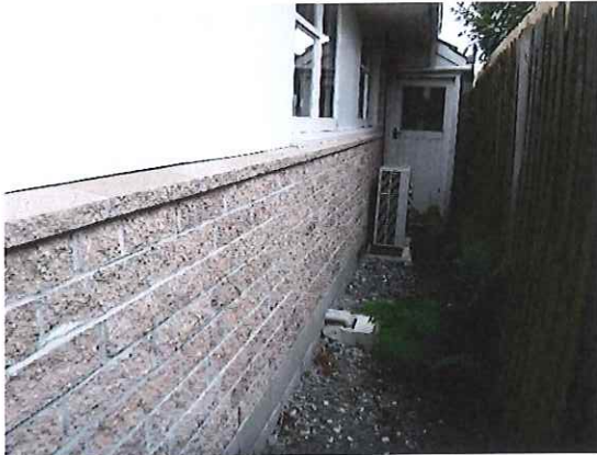
Photo 7. Re-cladded Summer hill stone and foundation block wall repair
