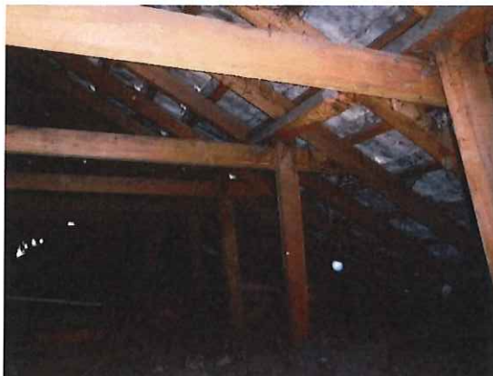
Photo 14. Roof space (View1)
