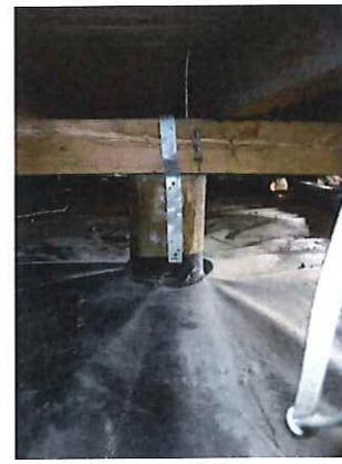
Photo 4. Steel strap connection to pile and bearer
