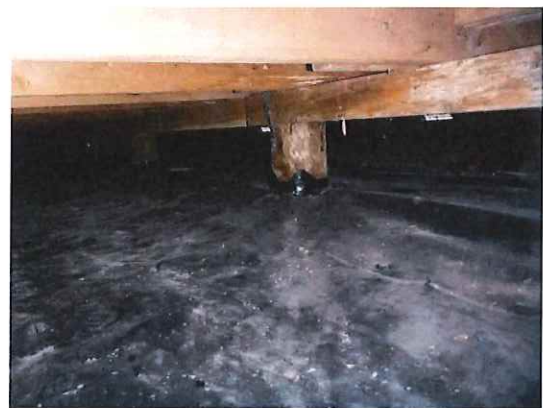
Photo 13. Sub floor space (View 3)
