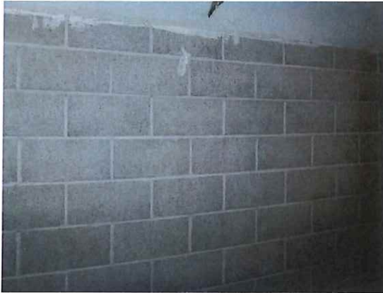
Photo 10. Garage concrete block wall from interior view.
