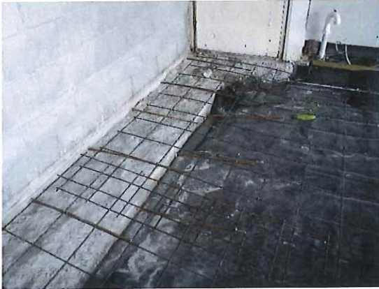
Photo 1. Garage concrete floor prior to pour concrete (View1)
