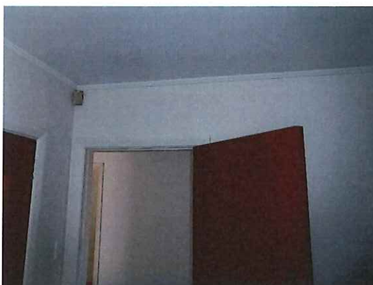
Photo 8. Dwelling wall lining and ceiling
