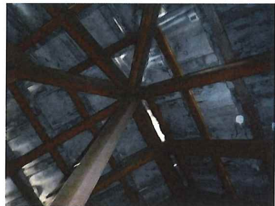
Photo 15. Roof space (View2)
