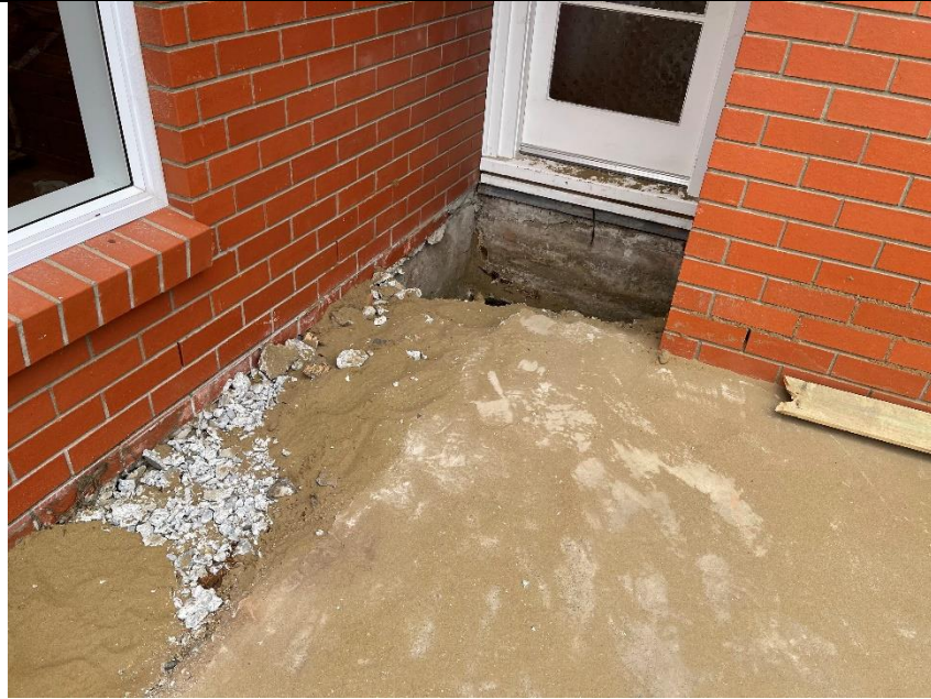
Photo 5 – Excavation under ring foundation for underpinning
