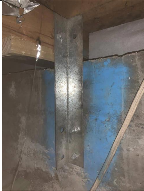
Photo 3 – Typical additional connections from concrete foundation to timber framing
