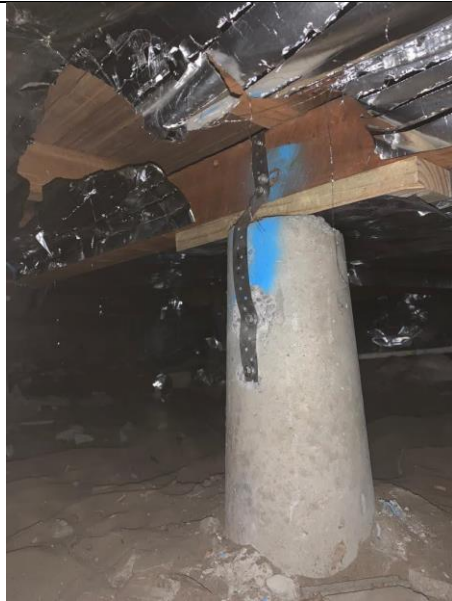
Photo 1 – Typical completed pile packing
