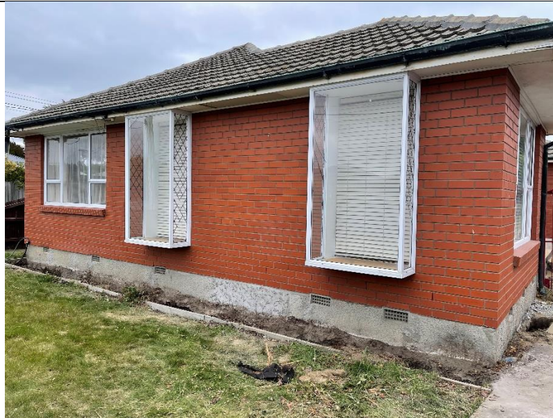
Photo 1 – Excavation under ring foundation for underpinning
