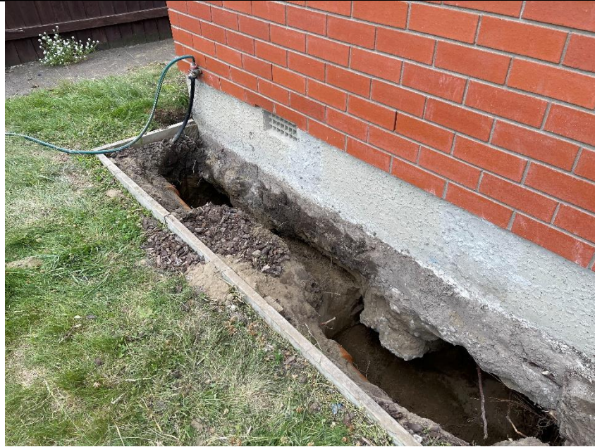
Photo 3 – Excavation under ring foundation for underpinning
