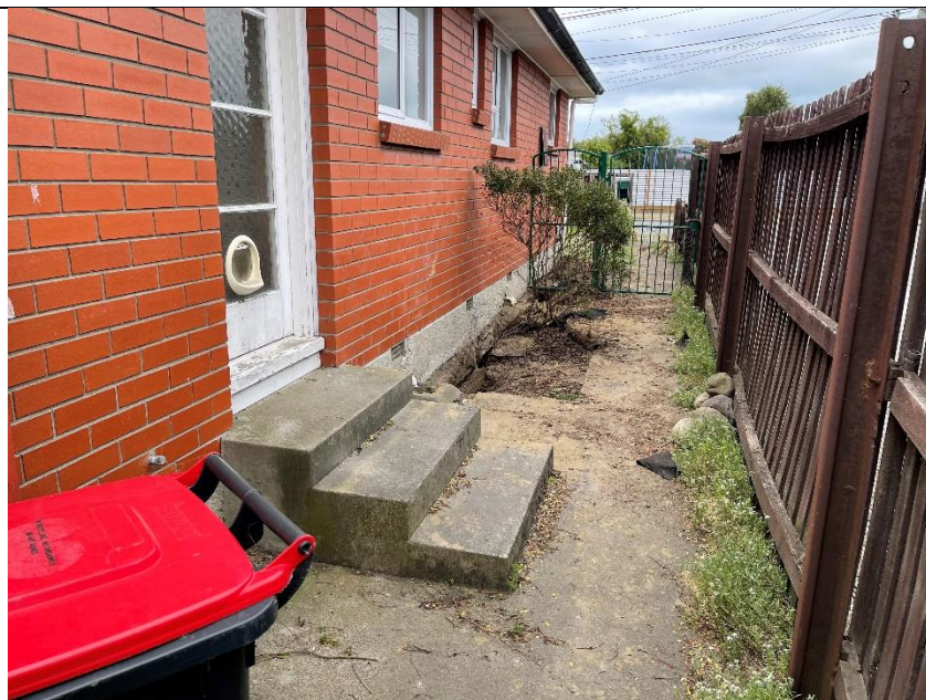
Photo 6 – Excavation under ring foundation for underpinning
