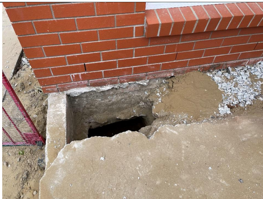
Photo 4 – Excavation under ring foundation for underpinning
