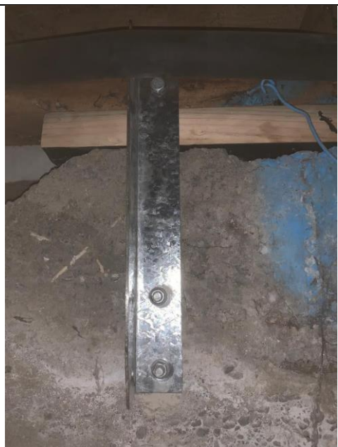
Photo 4 – Typical additional connections from concrete foundation to timber framing
