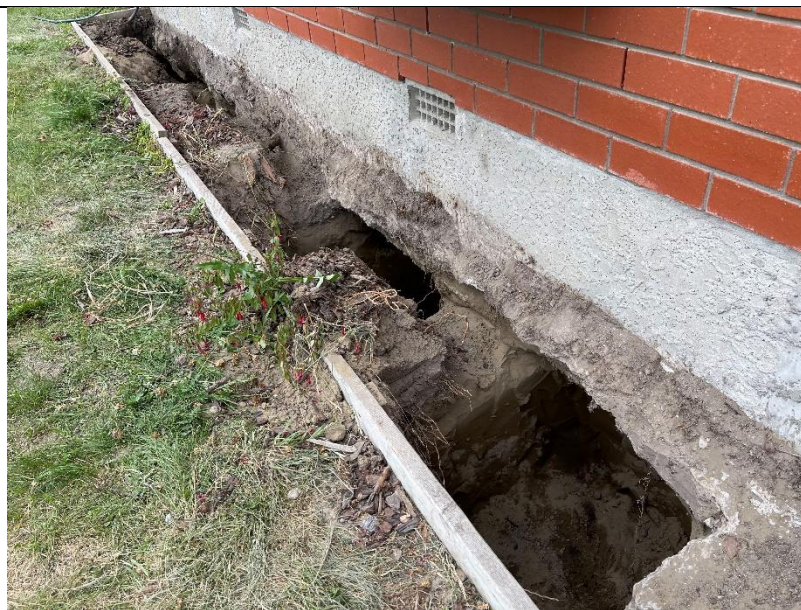
Photo 2 – Excavation under ring foundation for underpinning
