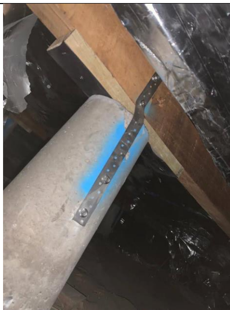
Photo 2 – Typical completed pile packing
