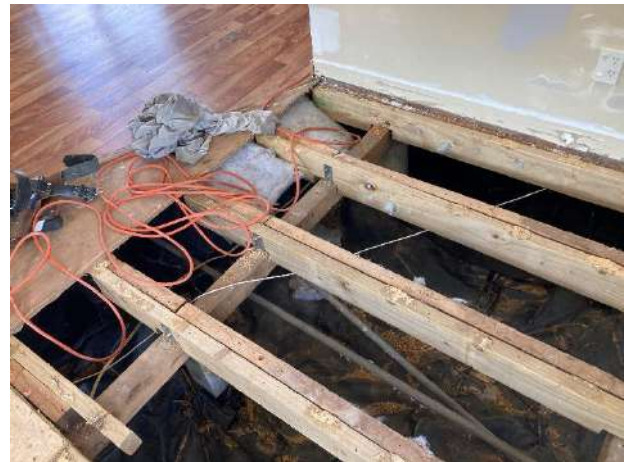
Figure 2 - fixings between joists and bearer.
