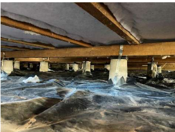
Figure 4 – New subfloor fixings in place, Packers are restrained
