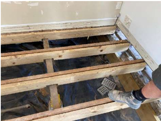
Figure 1 - Doubled joists is the area where floors heights are reduced – New plate can be seen along the foundation.
