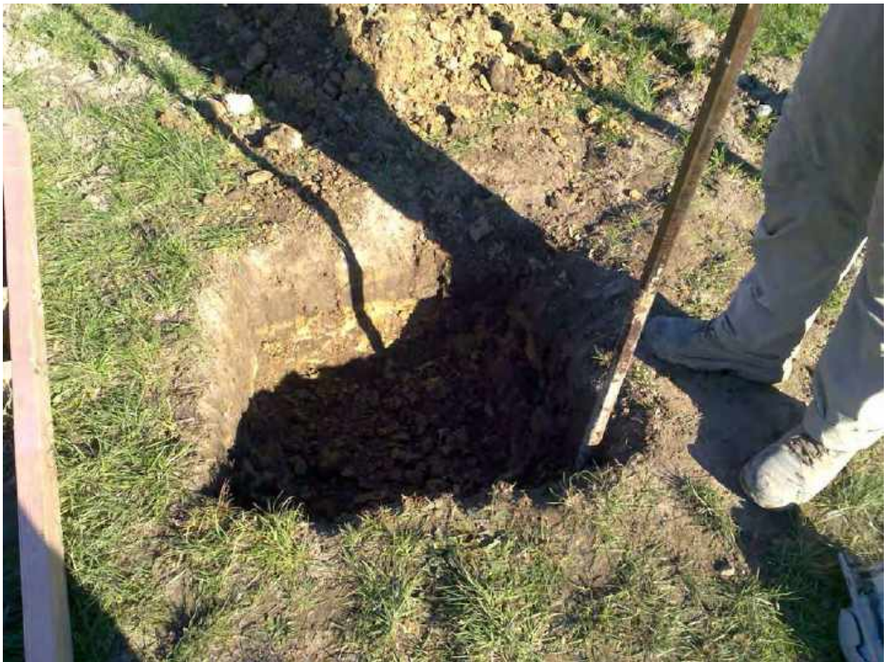
verandah hole being completed Taken at 2:44 PM on Wednesday 1/05/2019
