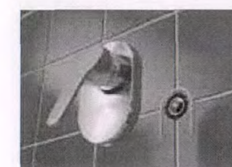
Run a bead of silicone sealant around the mixer unit on the tiles extending below the bottom of the pipe aperture.
