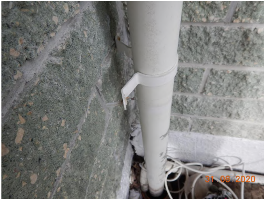
The bracket on the same downpipe has broken.
