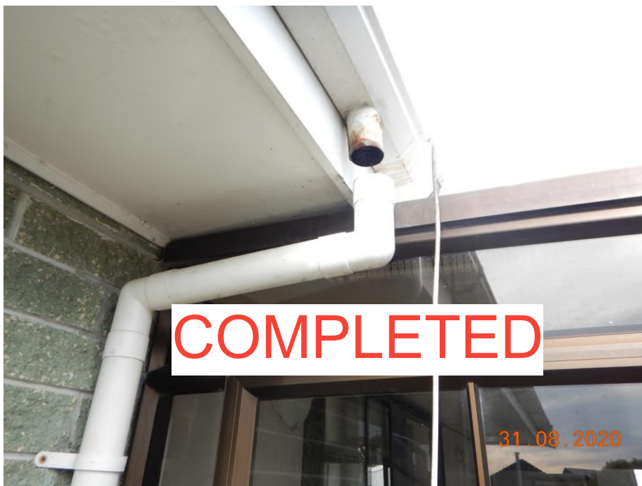
Downpipe is disconnected from the dropper.
