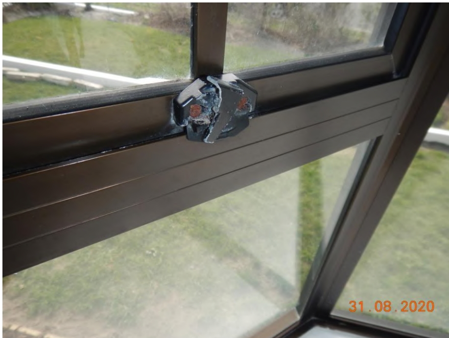
Broken window fittings can usually be easily replaced.
