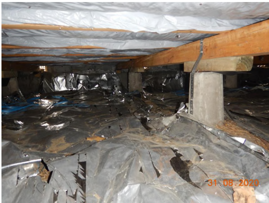
Sisalation cannot be repaired or replaced.
