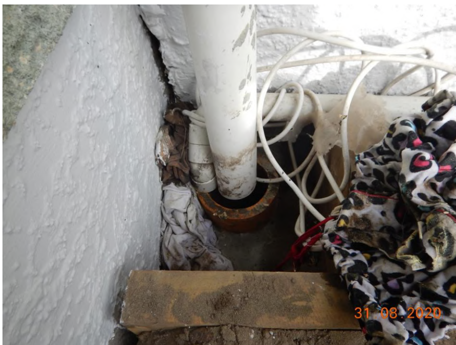
The smaller downpipe from the conservatory doesn't feed into the rise properly and will spill on the foundation, causing dampness and potentially undermining the foundation strength.
