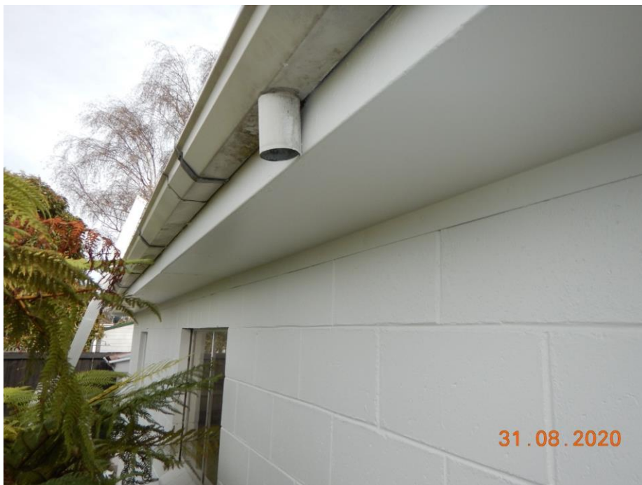
Dropper, but no downpipe and no stormwater riser, meaning no stormwater pipes to the garage.
