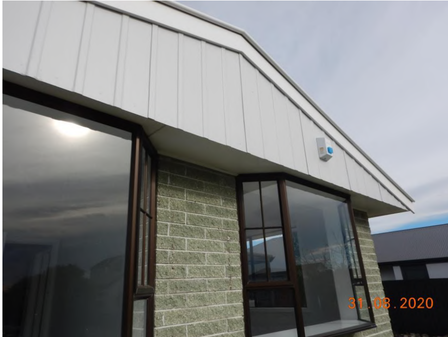
The profiled material of the gable and the flat soffit sheets may contain asbestos.
