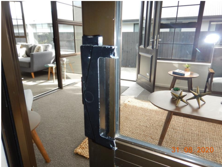
Broken door handle should also be able to be replaced.
