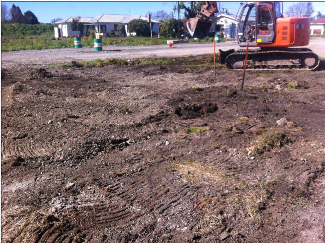
Photograph 4: View looking east at the footprint of the former agrichemical shed following the test pitting exercise.
