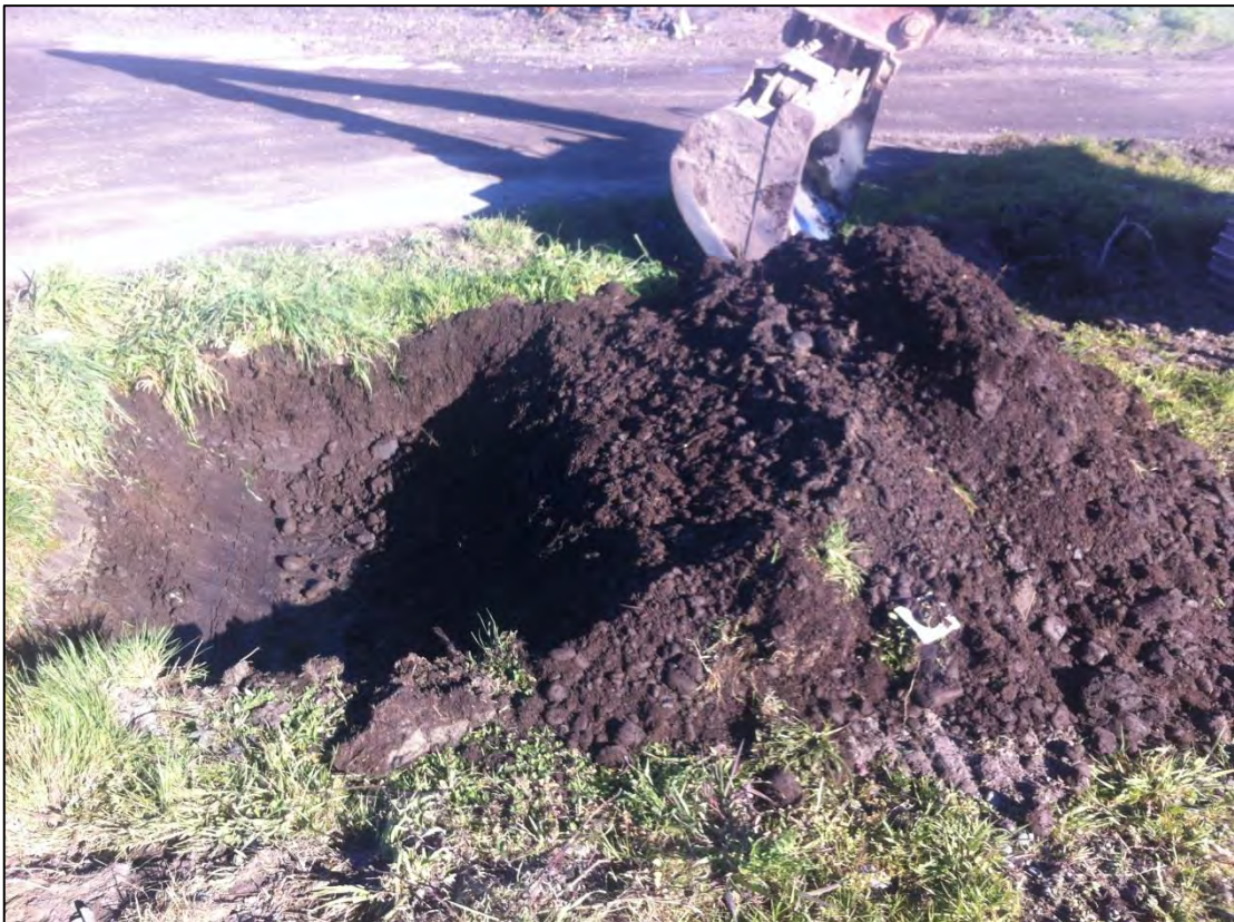
Photograph 2: View during the excavation of test pit CS6.
