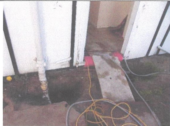
Exterior lifting pits – Sandy soils
