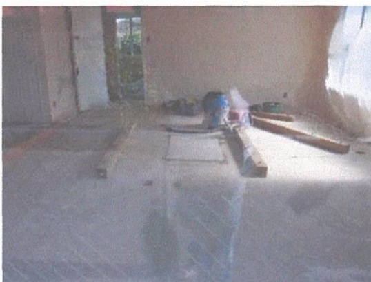
Interior lifting pits filled in but cracks not repaired yet.
