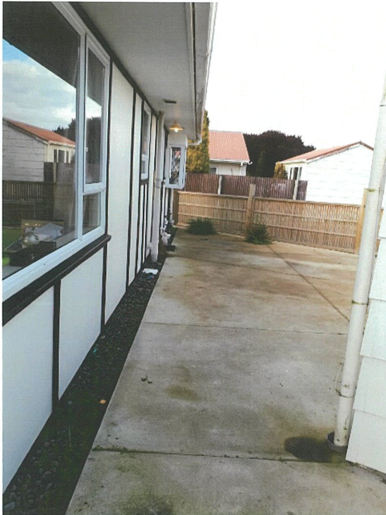
Figure 10 : West elevation. Concrete paths new since Canterbury events. Cracks to paths on all elevations, total replacement cost of damaged areas under excess of $5,000.00
