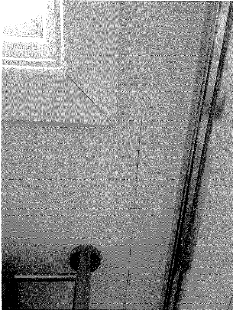
Figure 2 : Bathroom, crack to wall, window trim
