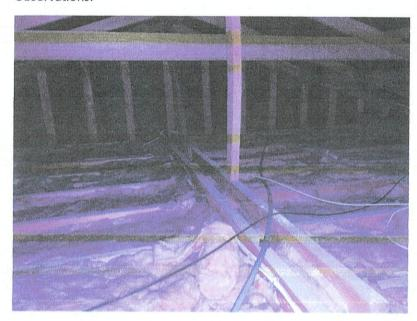
**Ceiling:** Existing insulation is Pink Batt ceiling insulation. The insulation is in good condition. The thickness is between 70mm and 80mm with good coverage. The approximate R-value is R1.4.
