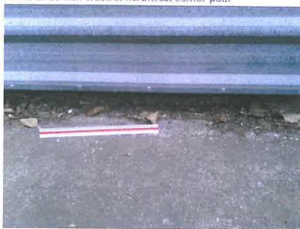
Photo 4: Garage slab 50 mm higher than driveway
