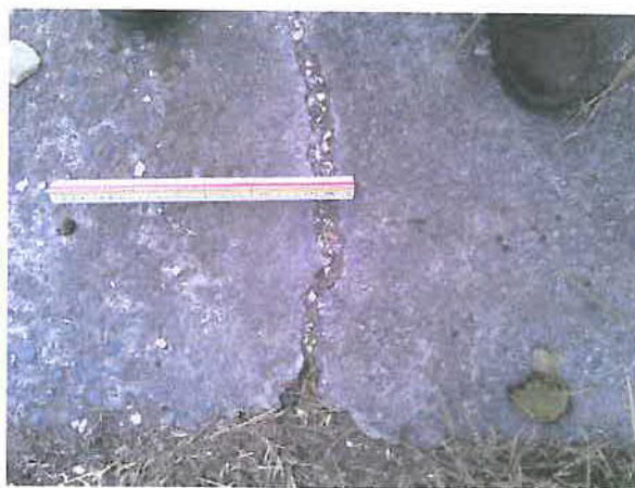
Photo 2: 30 mm crack in northwest corner path
