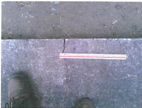
Photo 1: 5mm crack in northern path
