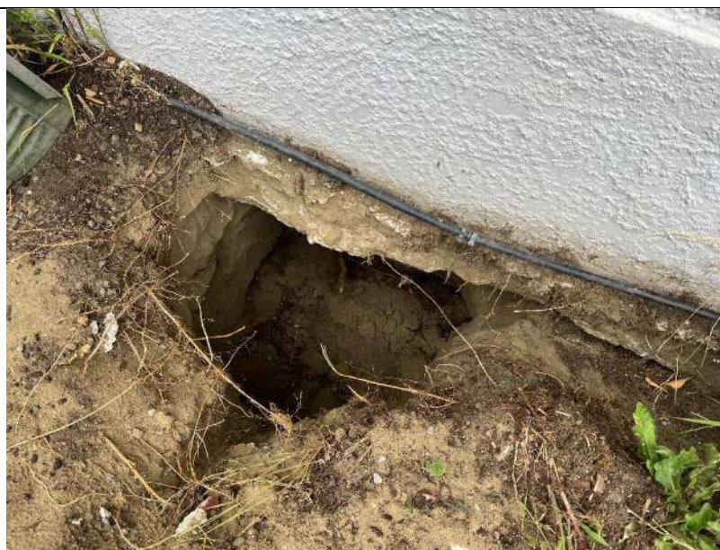
Photo 2 – Excavation under ring foundation for underpinning
