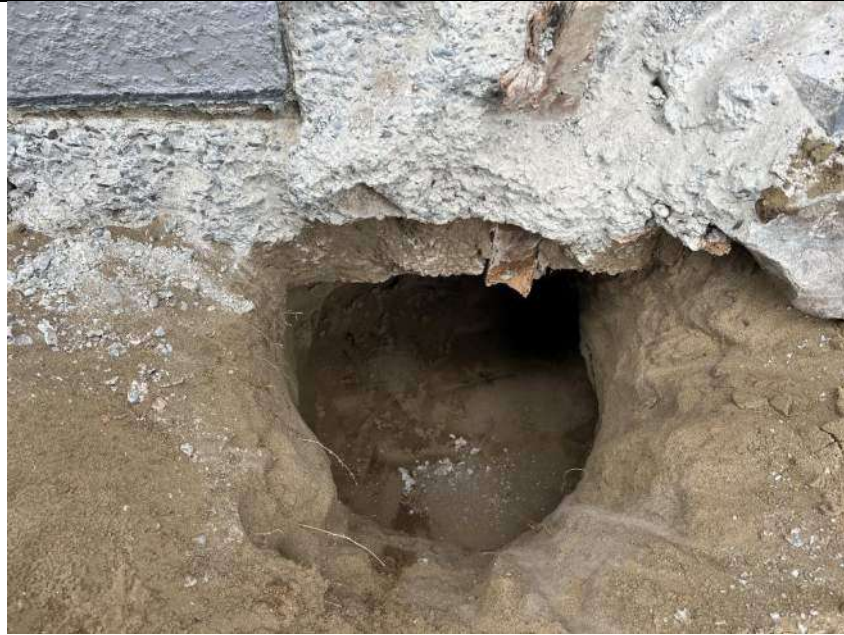
Photo 3 – Excavation under ring foundation for underpinning
