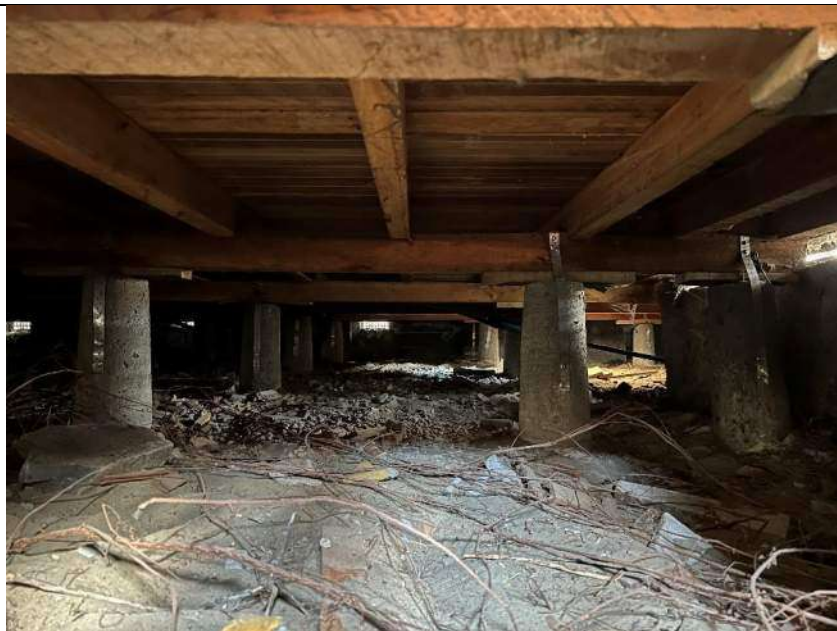
Photo 4 – Subfloor after jacking and packing
