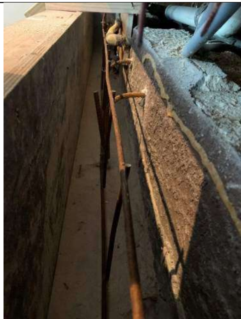
Photo 8 – Reinforcement installed for foundation beam thickening at extension junction
