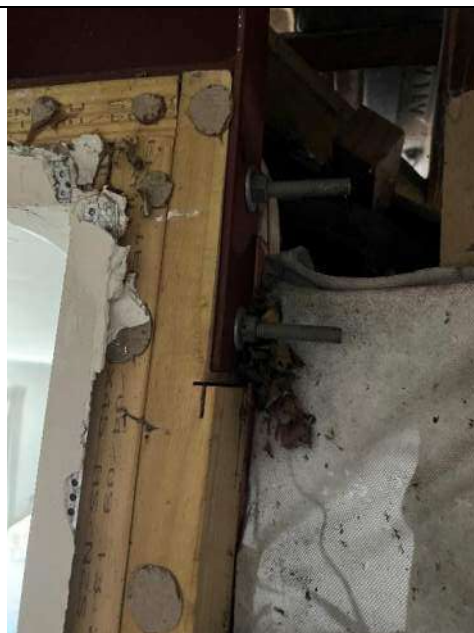
Photo 10 – Exposed steel beam connection to stud pack, steel beam connection is still in good condition with through bolts from steel end plate to studs.
