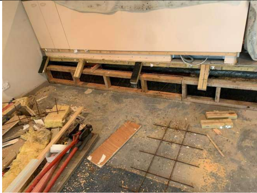
Photo 5 – Reinforcement installed for foundation beam thickening at extension junction
