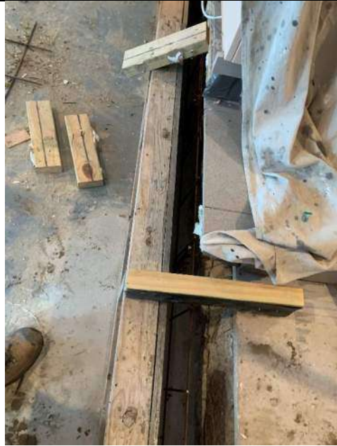
Photo 7 – Reinforcement installed for foundation beam thickening at extension junction
