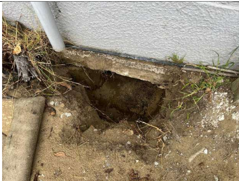
Photo 1 – Excavation under ring foundation for underpinning
