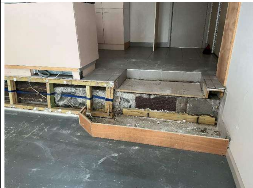
Photo 8 – Exposed concrete ring beam near the extension junction
