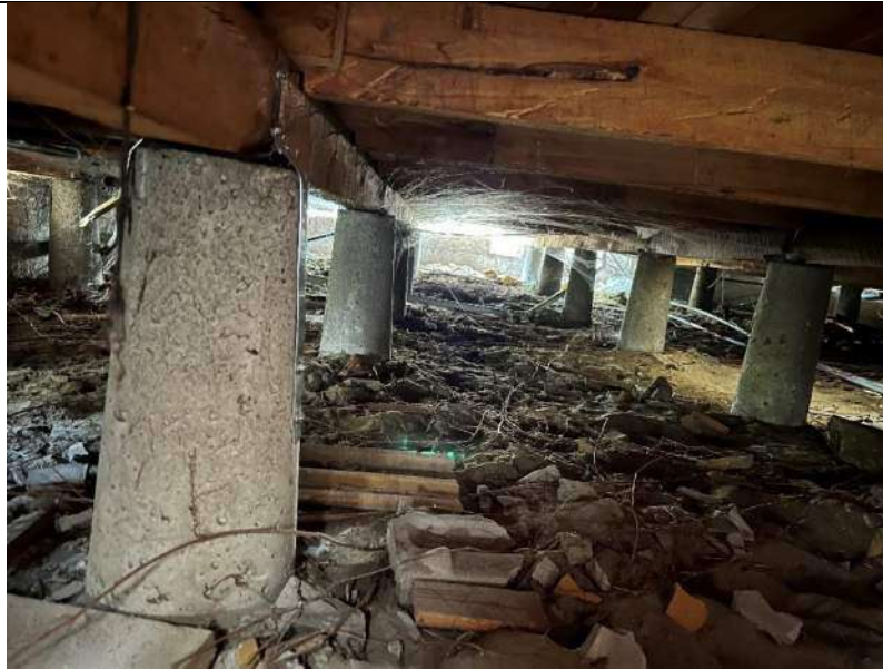
Photo 1 – Subfloor after jacking and packing
