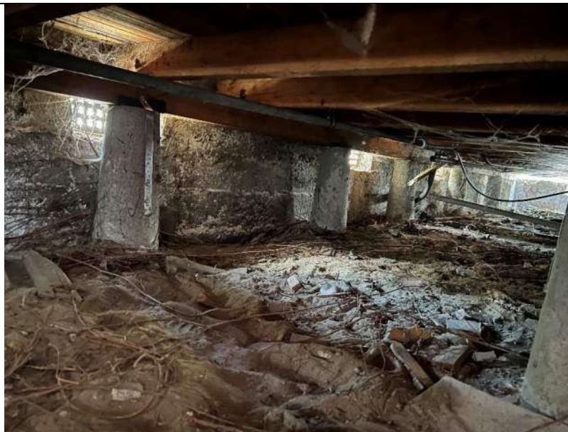
Photo 2 – Subfloor after jacking and packing
