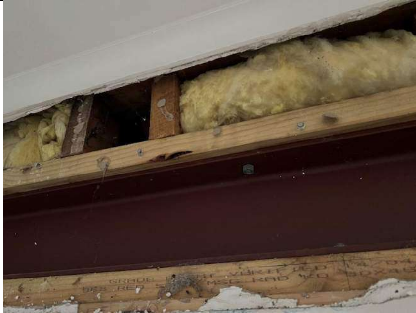
Photo 9 – Exposed steel beam above the kitchen
