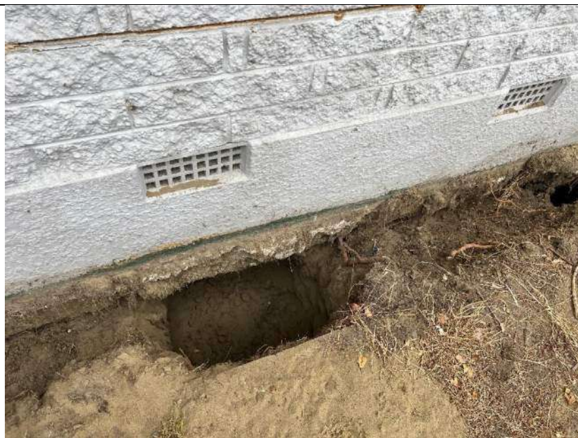
Photo 4 – Excavation under ring foundation for underpinning
