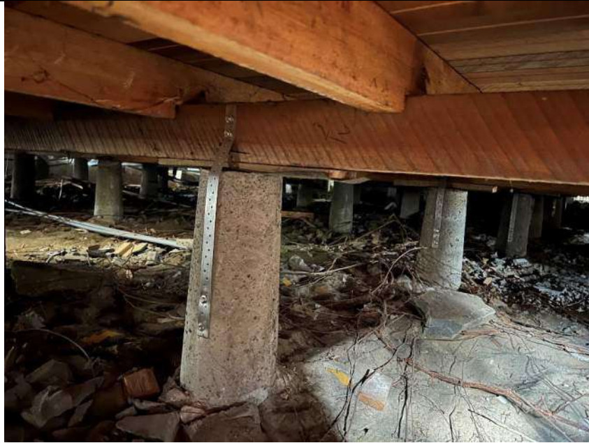
Photo 3 – Subfloor after jacking and packing
