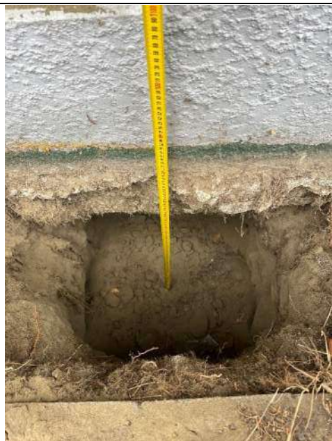
Photo 6 – Excavation under ring foundation for underpinning
