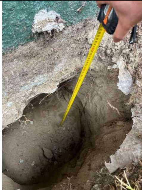
Photo 5 – Excavation under ring foundation for underpinning
