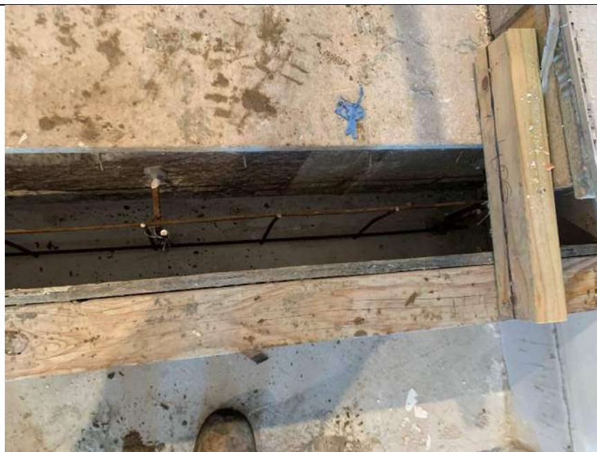
Photo 6 – Reinforcement installed for foundation beam thickening at extension junction
