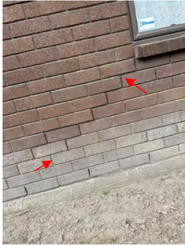
Mortar repair has re cracked slightly. This is only minor. One brick has a minor crack through it at the base.
