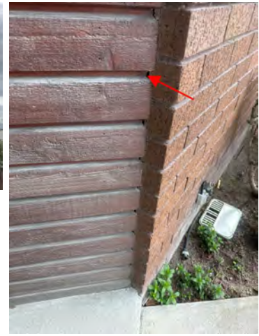
The gaps at this cladding transition could be filled to prevent moisture getting in these holes.
