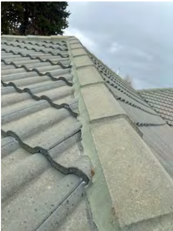
Cracking to mortar.
