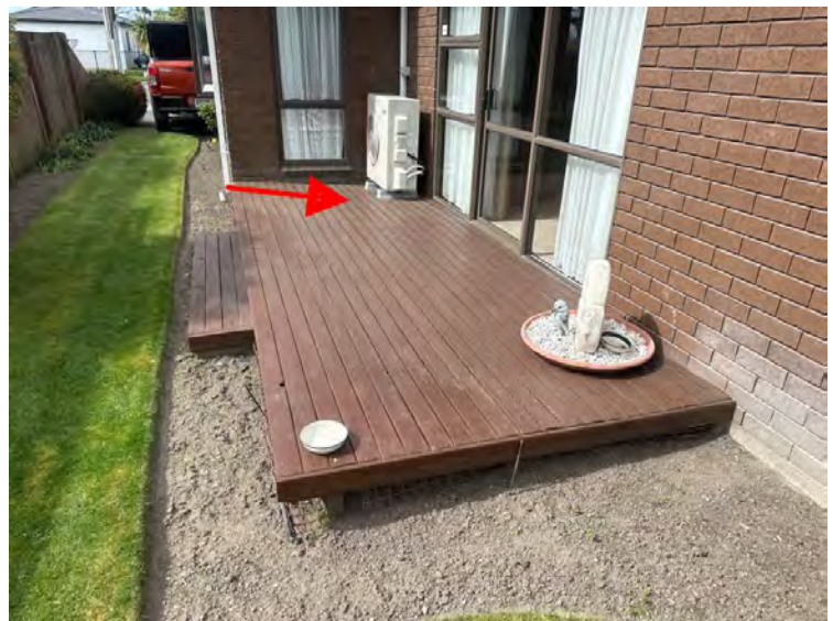
Deck looks to have sunk under the weight of the A/C unit. Extra support should be installed under this section of decking.
