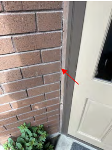
Install a facing at this transition to prevent moisture getting in here.
