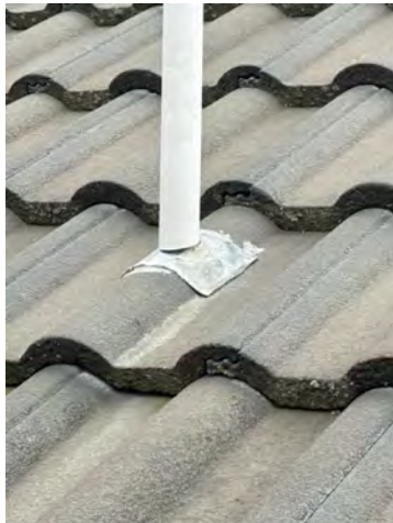
This flashing would benefit from a bead of sealant around it.
