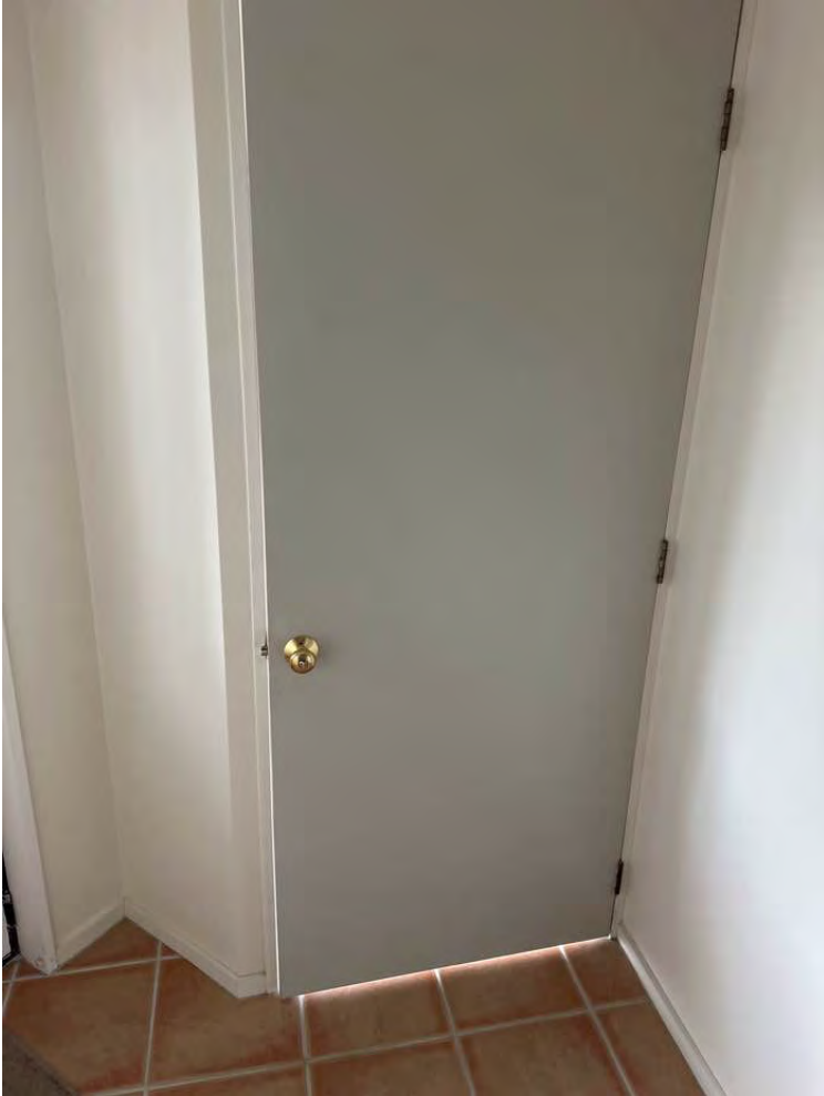
Internal garage door needs easing so it doesn't catch the frame.
