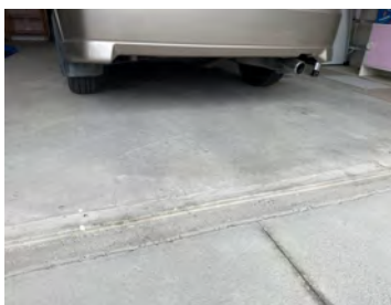
Minor hairline cracking to slab. Not concerning.
