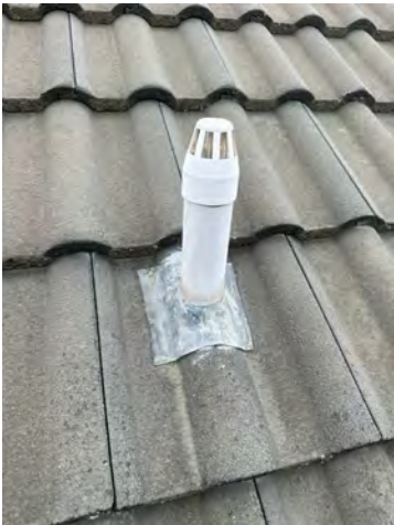
This flashing would benefit from a new bead of sealant around it.
