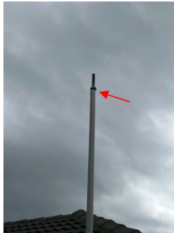
Push top cap on hot water boiler over pipe down.
