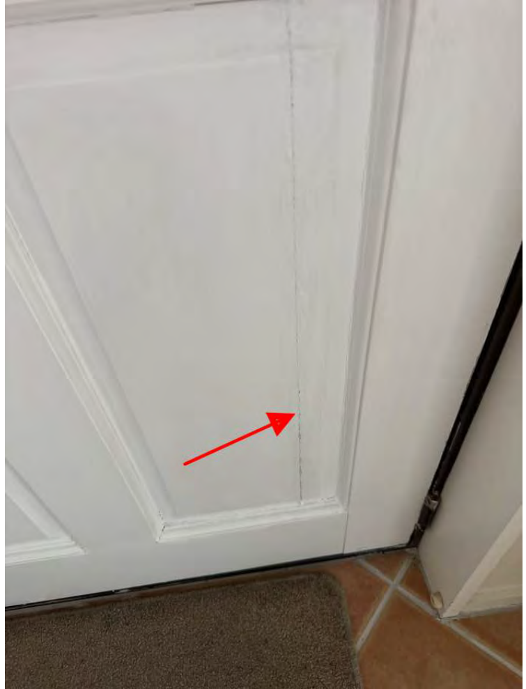
Front door has small crack in it.
