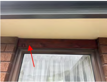
This board would benefit from new fixings to hold it back better.
