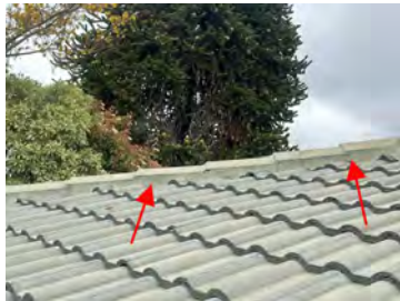
Cracking to mortar.
