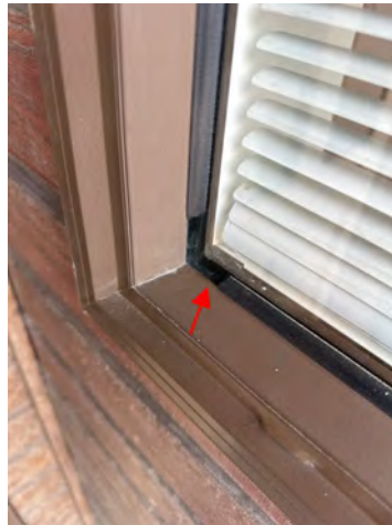
Example of rubber seals shrinking.
