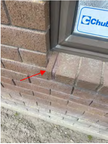
Slightly loose sill brick.
