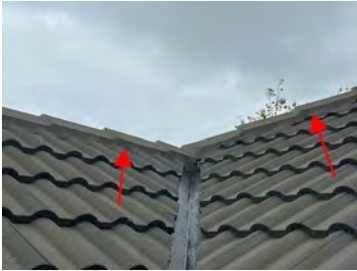
Minor cracking to mortar.
