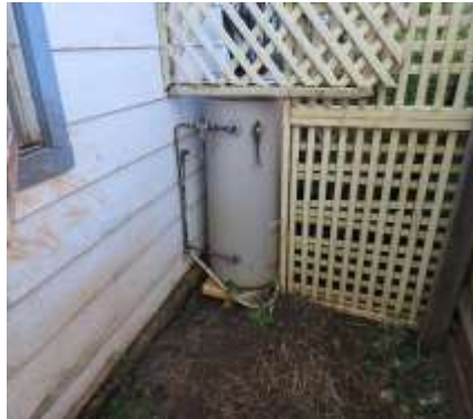
Electrical hot water system installed.
