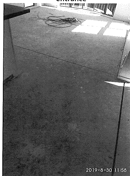
Fig 4: 20mm crack in living area
