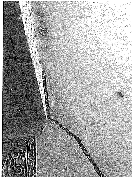
Fig 2: Cracks in the pavement – near the entrance
