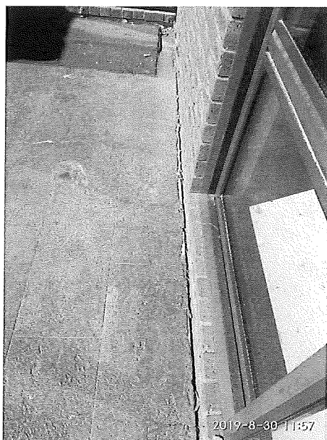
Fig 3: Crack in concrete block southwest of the house
