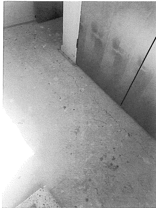
Fig 6: Crack in room 3(refer to Procerto drawings)
