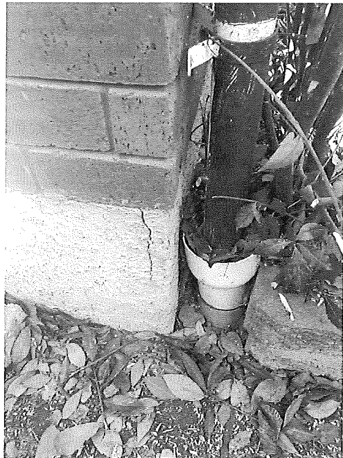
Fig 7: Crack in perimeter foundation
