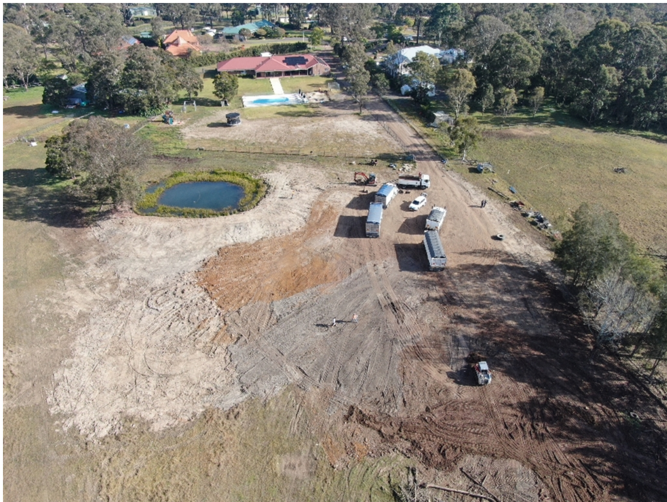
Image Two: Depicting the extent of the fill material at the Premises which has been land applied and spread at the Premises.
