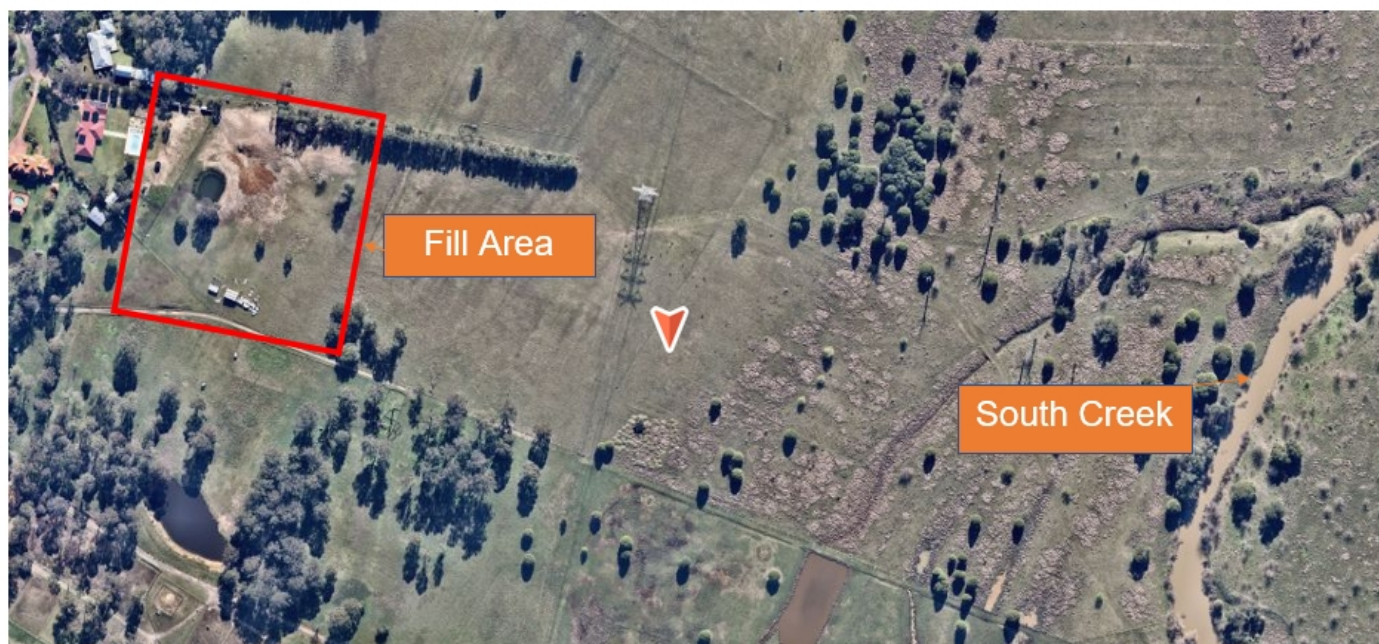
Image Three: Depicting proximity of contaminated waste material at the Premises to South Creek.
