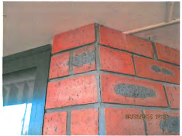
Figure 6: Crack in mortar joints of brick
