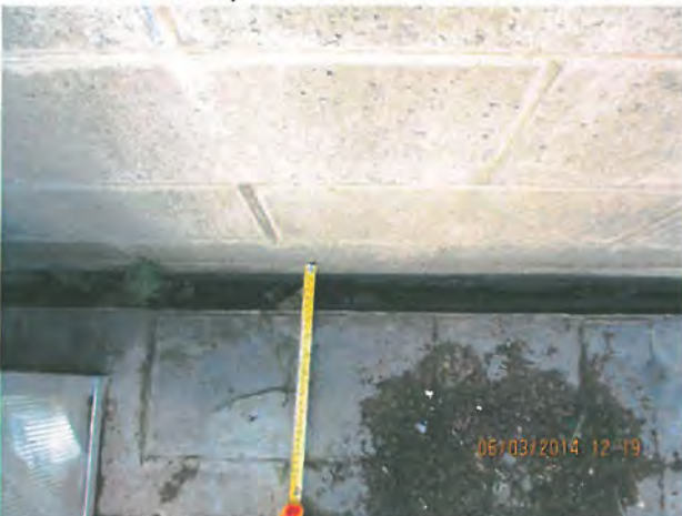
Figure 6: 65mm gap between paving and garage
