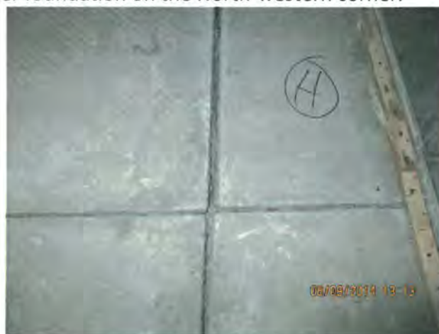
Figure 2: Construction Joints have opened
