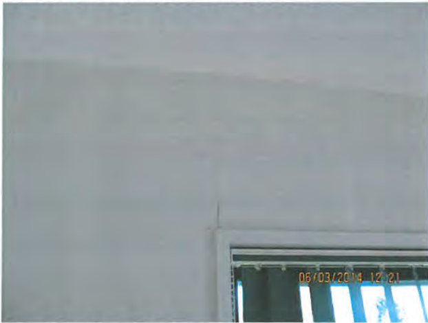
Figure 5: Minor damage to wall linings
