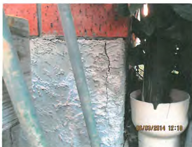
Figure 3: Crack in perimeter foundation
