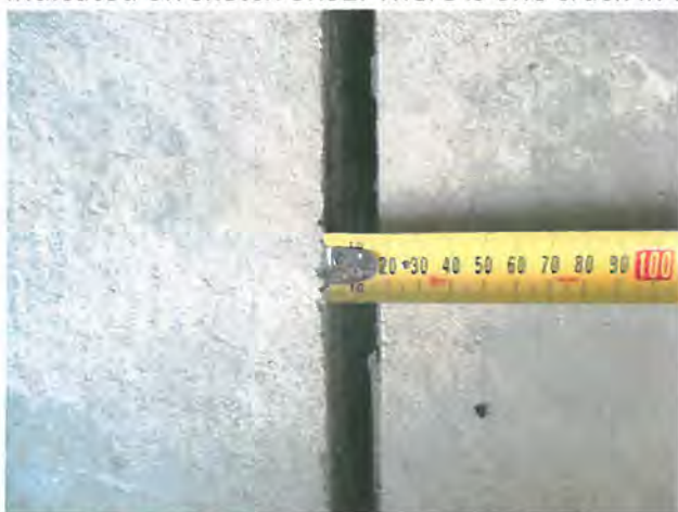
Figure 1: Construction Joint Separated 18mm
