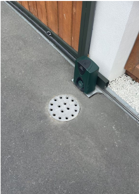
Surface Water Control: Working Condition In Order
