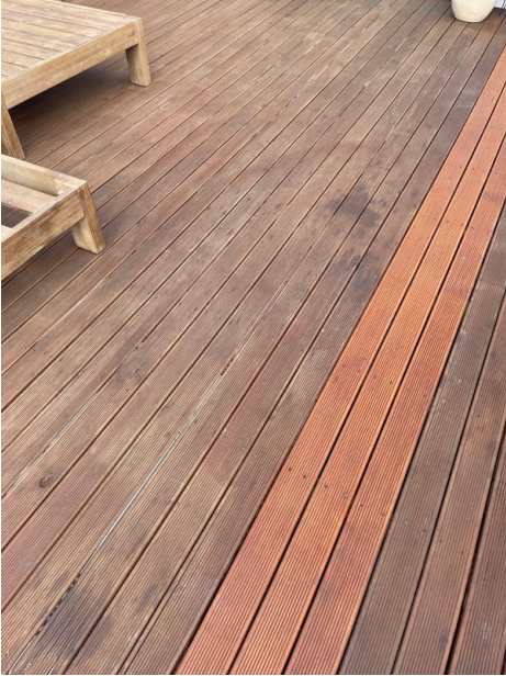
Decking: Material Timber
