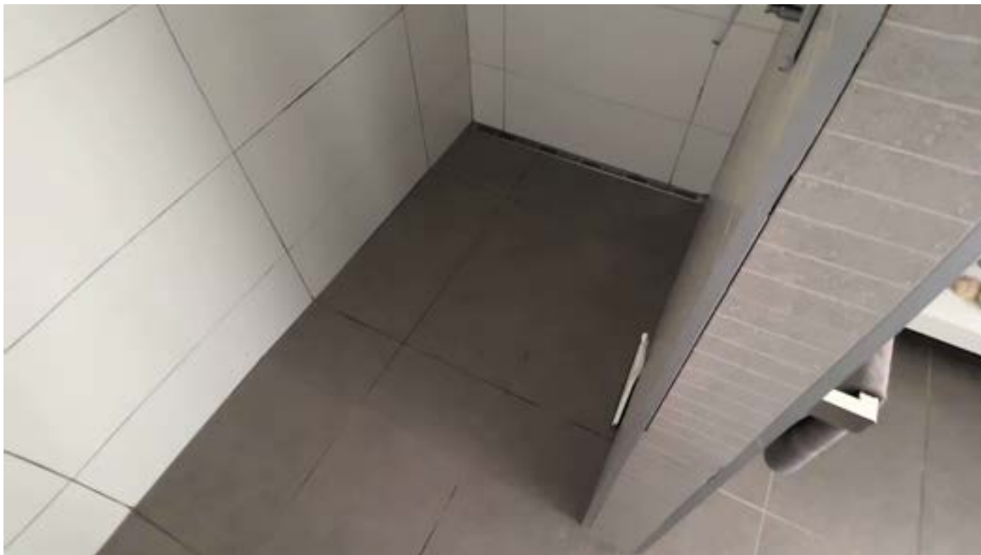
Main bathroom shower
