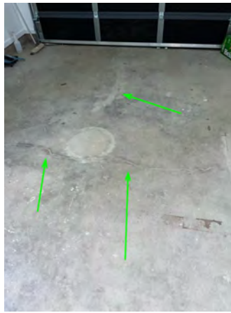
Cracks in the floor slab that have been repaired.
