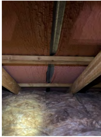
Example of the roofing paper shrinking with gaps in the underlay.
