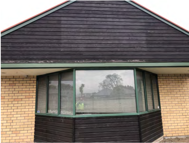
Shiplap weatherboards look sound but need restaining.
