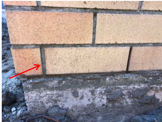
2 Minor Gap in mortar to rake & replace mortar
