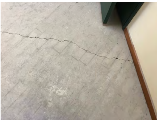
1: Minor Crack in concrete Floor to V out & epoxy fill.
