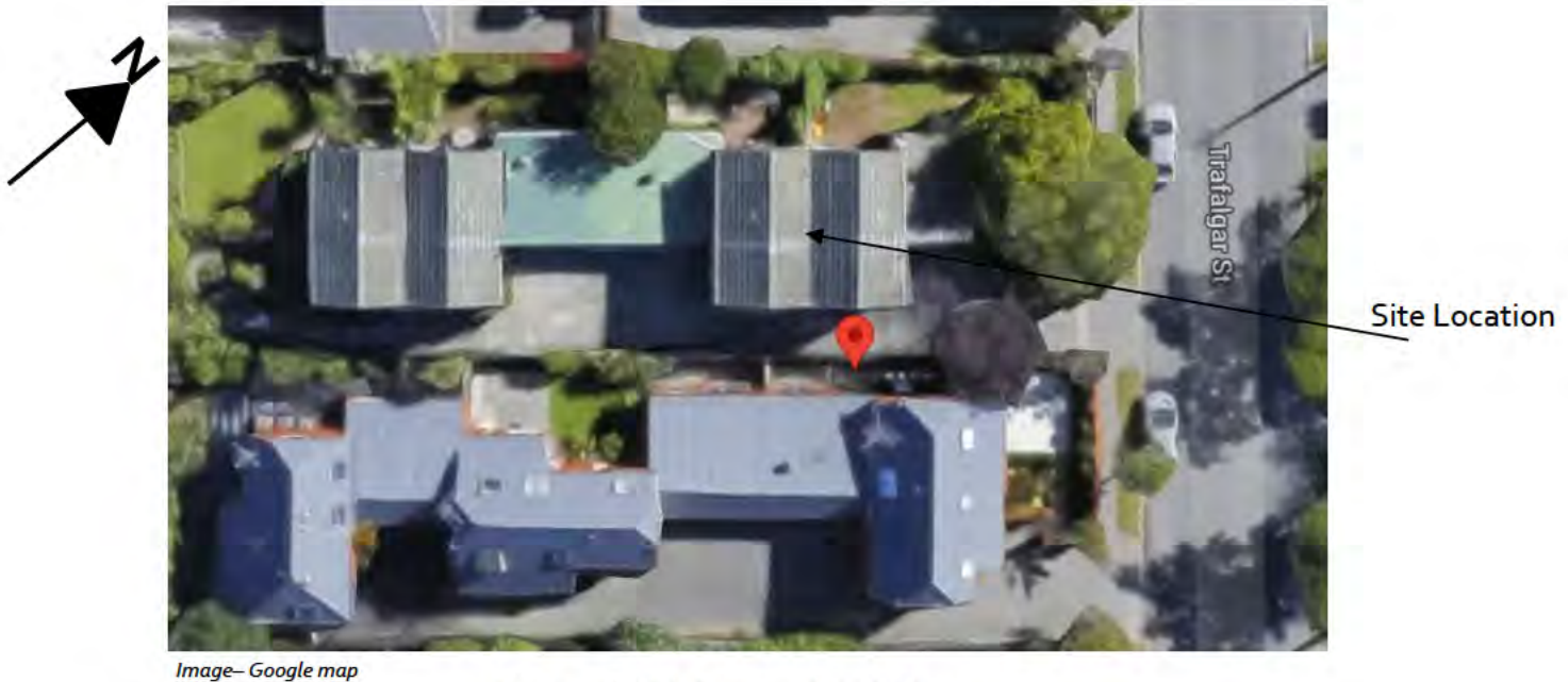
Figure 1. Aerial photograph & site layout.
