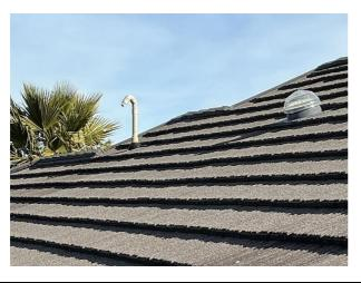
**Photo 8**East side heater and skylight penetrations.
