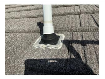
**Photo 6**North side vent penetration.
