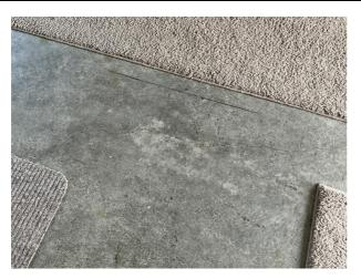
**Photo 19** Crack in the garage slab, no issue.
