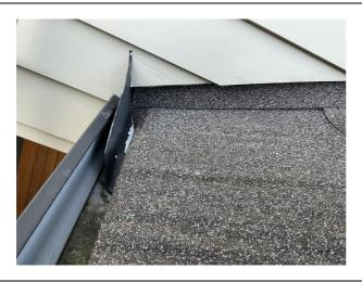
**Photo 4**Roof and wall junctions are fitted with a kick out diverter flashing.
