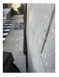
**Photo 68**North side vent pipe has moved away from the house with the path.
