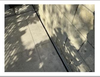
**Photo 56**Gaps visible between the path and house.
