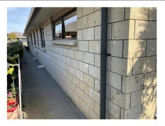
**Photo 15**No issues with the brick veneer.
