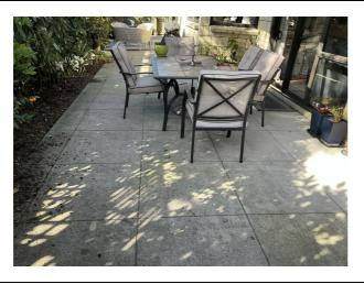
**Photo 55**North side has settled on the boundary side
