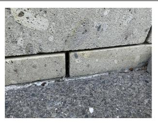
**Photo 17**Weep holes are present throughout the brick work.
